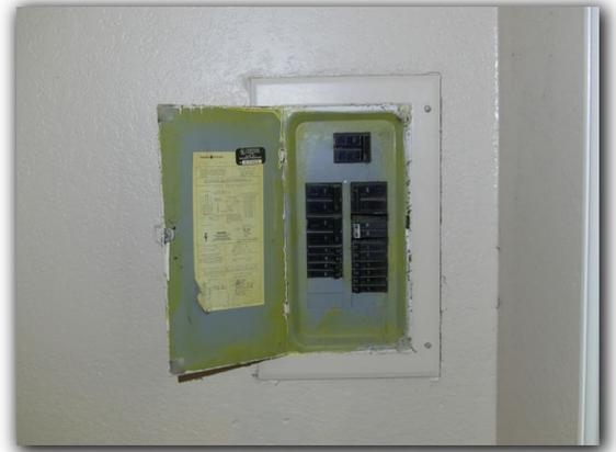
The electric service panel breaker use was not labeled. Each electric service panel breaker should be adequately labeled as to what appliance or circuit it serves.
