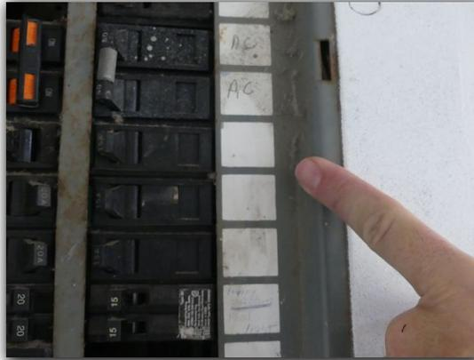
The electric service panel cabinet cover plate or dead-front screws were observed to be sharp (SAFETY HAZARD) and should be replaced with the proper screws.
