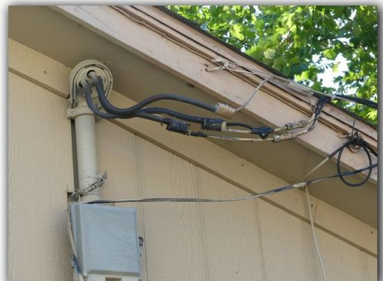
☑ The overhead service drop electrical conductors had inadequate clearance from tree branches.
