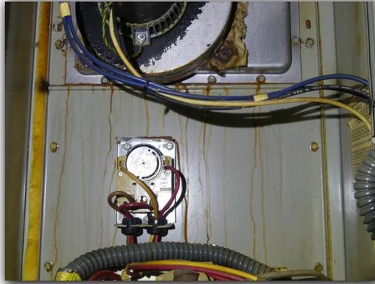
Older style gas valves require a tool to operate at the heating equipment. Under current building standards, gas valves should be operable by hand.
