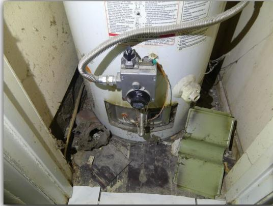
Corrosion and / or signs of an intermittent water leaks were observed at the water supply valve or water heating equipment plumbing connections. Water leaks and corrosion at the water heating equipment may cause water damage and should be repaired or replaced as needed by a certified, licensed water heating equipment specialist.
