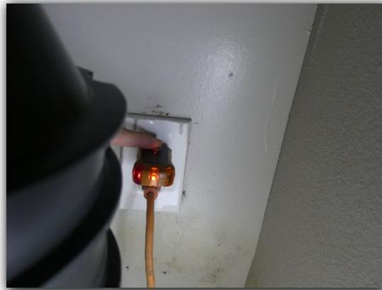
The refrigerator electrical receptacle was observed to lack ground fault circuit interrupter (GFCI) device protection. According to the 2014 NEC electrical standards, refrigerator electrical receptacles should be GFCI protected. Lack of GFCI protection in required locations is a SAFETY HAZARD.
