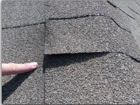
Additional sealants were installed at the roof covering materials or flashings. Added sealants may be an indication of previous repairs, water intrusion, improper installation or other defects.
