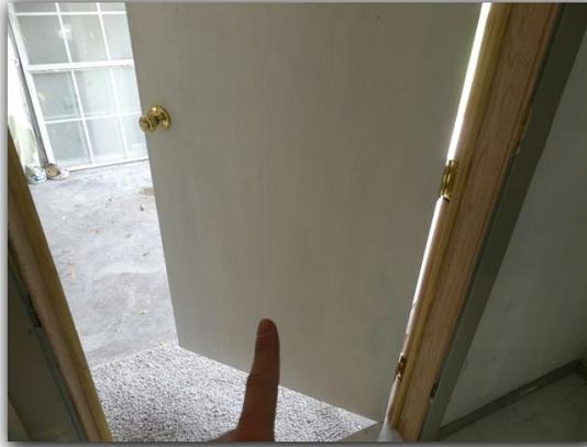
The garage entry door was observed to have damaged weather stripping. Under current building standards, the entry door between the garage and the residence should be well sealed to prevent vehicle storage area fumes from penetrating the structure. Lack of an airtight garage entry door is a SAFETY HAZARD.
