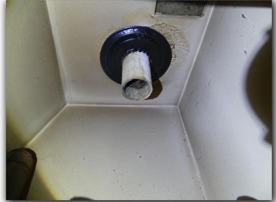
The gas-fired water heating equipment was not properly vented for combustion and dilution air. Improper ventilation at the gas water heating equipment was observed to be a SAFETY HAZARD and may allow unwanted vapors to accumulate. Improper gas water heater ventilation may affect water heater performance. Further evaluation is recommended.
