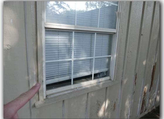
The window above the tub/shower did not appear to have a safety glass etching or label. Glass less than 5' above the tub/shower should be tempered safety glass. Lack of safety glass in required locations is a SAFETY HAZARD and should be replaced.
