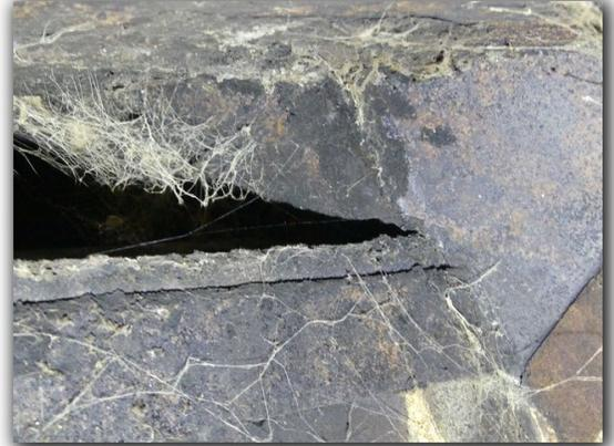
The fireplace firebox brick and or brick mortar have been damaged. Damaged firebox brick or mortar may allow heat to transfer to flammable materials and is a SAFETY HAZARD that should be repaired by a qualified fireplace specialist.
