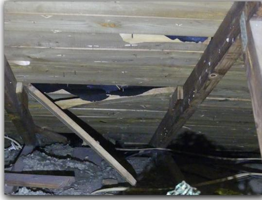
Openings were observed in the attic at electrical, plumbing, duct work or other penetrations where they pass through structural framing. These opening should be sealed for improved FIRE SAFETY.
