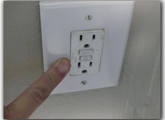
Electrical receptacles, switches and or covers were observed to be loose, damaged, missing or missing screws and were in need of repair. Damaged or missing electrical receptacles or switches should be repaired by a certified, licensed electrical specialist.
