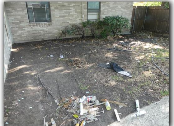
High soil levels were observed at the foundation/brick line. 4 to 6 inches of the foundation perimeter beam should be visible. High soil levels may block weep holes and prevent proper wall ventilation. High soil levels create conducive conditions for wood destroying insects and water intrusion. High soil levels prevent the inspector from observing the foundation perimeter beam. Correction of inadequate grading clearance to exterior wall and foundation surfaces is recommended.
