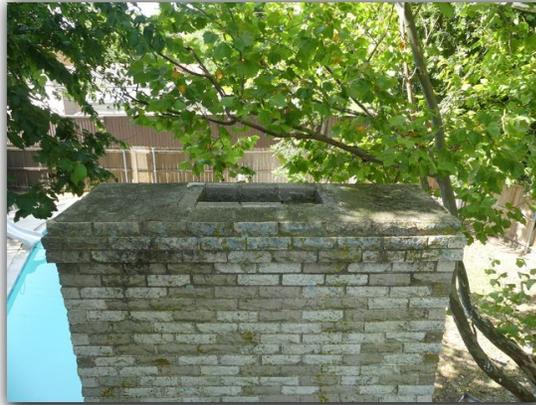
A damaged or missing chimney spark arrester was observed to be a SAFETY HAZARD and should be repaired or replaced by a qualified chimney specialist.
