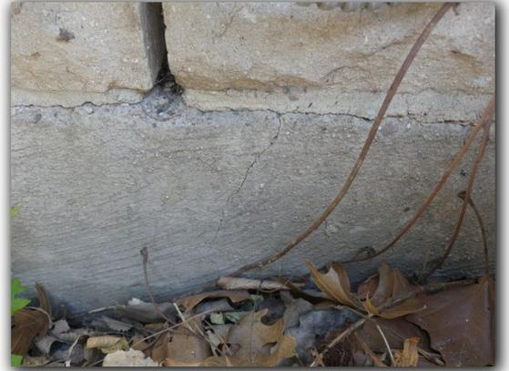
Exposed or damaged metal foundation reinforcement components were observed. Exposed or damaged metal foundation reinforcement components may lead to additional foundation deterioration and adverse foundation performance. This condition should be repaired as needed by a foundation specialist.
