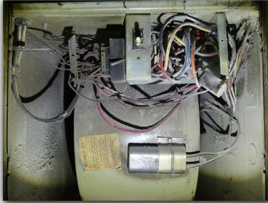
Signs of rust or corrosion were observed at the heating equipment. Rust, corrosion or discoloration may be indications of age, wear, lack of maintenance or other defects. The heating equipment should be further evaluate by a certified, licensed heating equipment specialist and repaired or replaced as needed.
