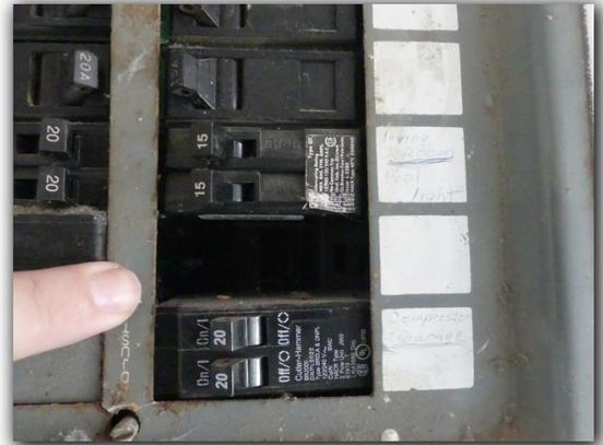
Double tapped breakers were observed to be a SAFETY HAZARD in the electric service panel. Each breaker should provide electric service to only one circuit. The inspector recommends that the electric service panel be further evaluated and repaired or replaced as needed by a certified, licensed electrician.
