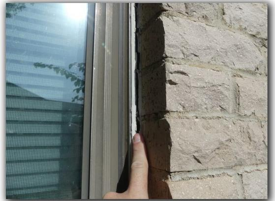
The window weather-stripping was observed to be damaged. Damaged or missing weather stripping around windows may allow moisture penetration, conditioned air loss and insect penetration and should be repaired.
