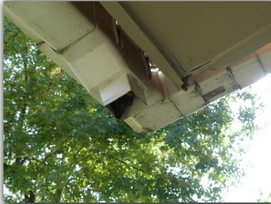
The gutters and downspouts contained leaves and other debris and should be cleaned out to allow for proper drainage.
