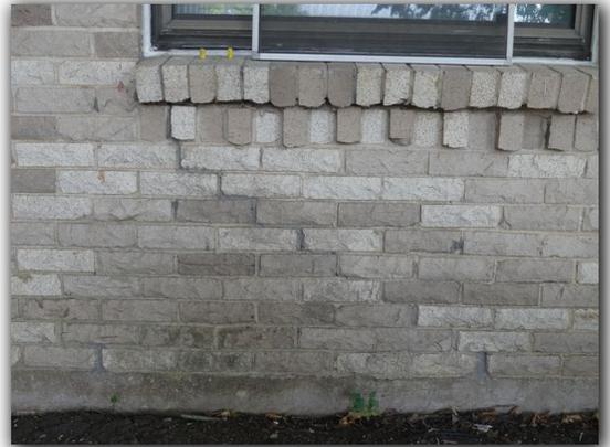
Mortar is damaged, separated or missing in one or more areas. Missing, separated or damaged exterior masonry mortar may allow moisture penetration and should be repaired.
