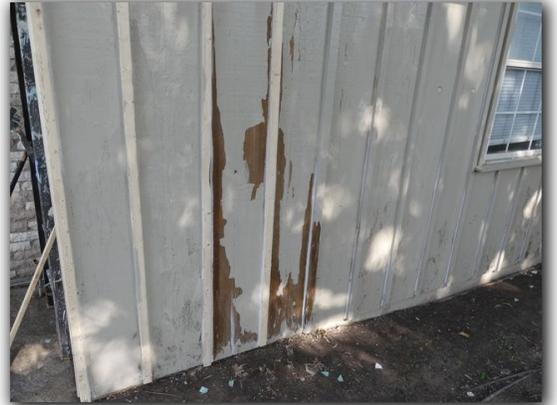
Peeling, damaged or deteriorating paint, stain and/or sealant was observed at the exterior trim. Peeling, damaged and deteriorating paint or sealant should be repaired to prevent moisture penetration and deterioration of materials.
