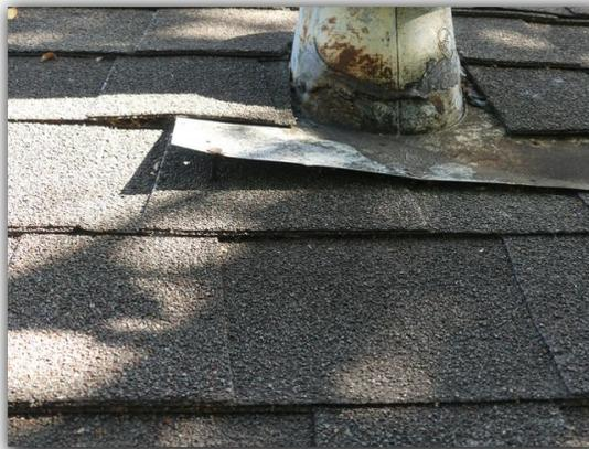
Leave, sticks, branches and other debris were observed on the roof covering and may contribute to roof covering material damage and water penetration. The roof covering surfaces should be free of leaves, sticks, branches and debris.
