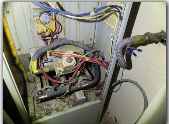
There were gas fired appliances that did not have a "drip leg" installed. Under current construction standards, drip legs are required at the black iron gas pipe prior to a flexible gas line connection.
