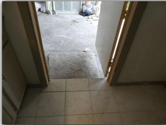
The garage entry door was observed to be a non-fire rated door. Under current building standards, the entry door between the garage and the living area should have a minimum of a 20-minute fire block rating for improved FIRE SAFETY. Lack of a fire rated garage entry door is a SAFETY HAZARD.
