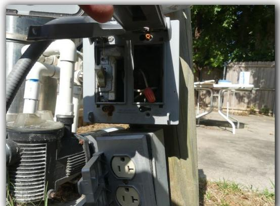
Lack of bonding at pump motor, water heater, blower, or other electrical equipment to ground was observed to be a SAFETY HAZARD. Inadequate electrical bonding should be further evaluated by a qualified specialist.
