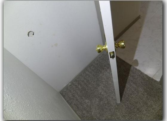
Interior doors which are in contact with the floor covering should be repaired. Door which are in contact with floor covering may damage the flooring.
