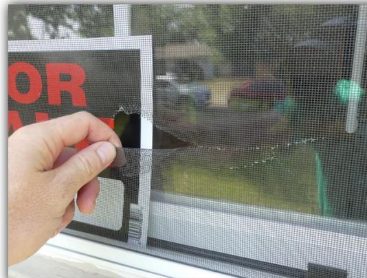
Windows were observed to be missing window screens. Window screens help protect window glass from minor impact damage and prevent insect penetration at the windows. Missing window screens should be replaced.
