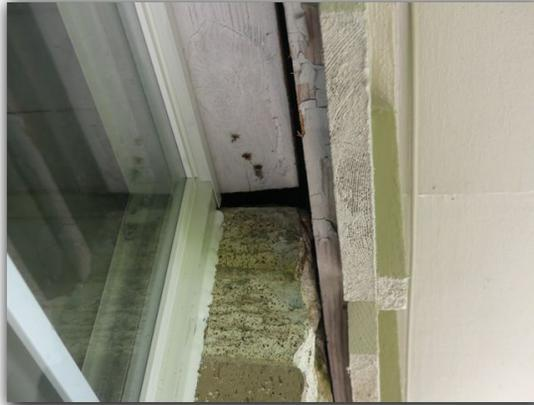
Weep holes were not open, were missing and/or were improper spaced at the lower brick/stone of the exterior walls. Weep holes should be installed and properly spaced to provide proper wall ventilation.
