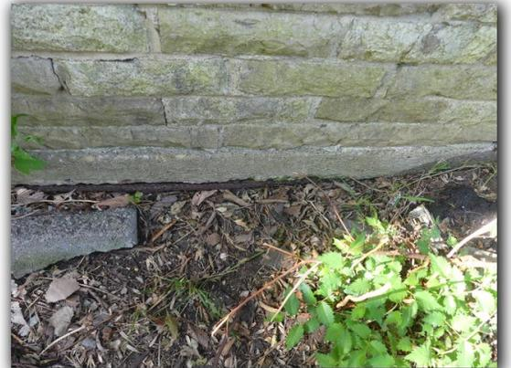
Foundation slab corners have been sheared off (corner pop). This is a common condition in slab on grade foundations and should be repaired. Repairing corner pops is recommended to prevent moisture and wood destroying insect penetration.
