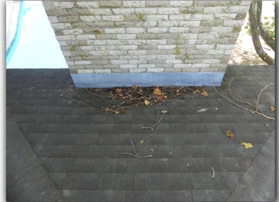
The tree branches within 10' of the chimney were observed to be a SAFETY HAZARD and should be removed. Flammable materials such as tree limbs should not be within 10' of the chimney for reasons of safety.
