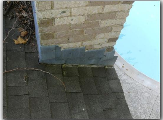
Exposed nail heads were observed at the roof coverings. Exposed nail heads may allow water penetration and were in need of repair.
