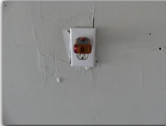
Open ground connections were observed at electrical receptacles. Open ground electrical receptacles are a SAFETY HAZARD and may cause damage to modern electric appliances. The cause of open ground electrical receptacles should be determined and repaired or replaced as needed by a certified, licensed electrical specialist.
