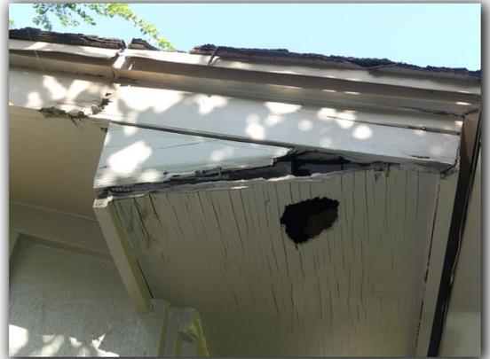
Damaged or missing attic gable vents or vent screens should be repaired to prevent wildlife penetration and other defects.
