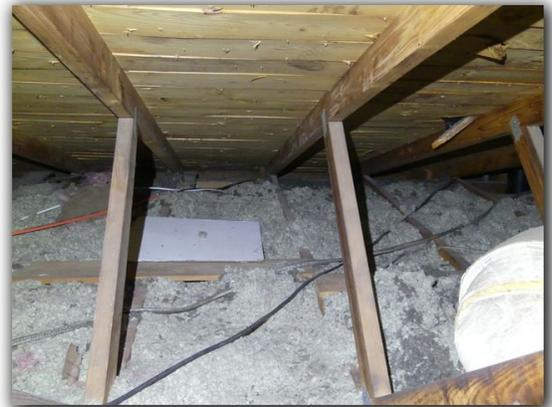
Water stains were observed on the roof sheathing (decking). The cause of the water stains should be determined. You are strongly encouraged to have your insurance company and a certified, licensed roofing contractor to physically inspect the roof covering materials, prior to closing, to fully evaluate the insurability and condition of the roofing material.
