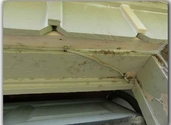
Improperly terminated electrical conductors were observed. All electrical conductor connections should be installed in sealed junction boxes for reasons of safety. Improperly terminated electrical conductors should be repaired by a certified, licensed electrical specialist.
