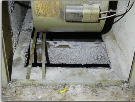
The cooling equipment showed signs of being dirty. Cleaning, servicing and / or further evaluation by a licensed professional is recommended.
