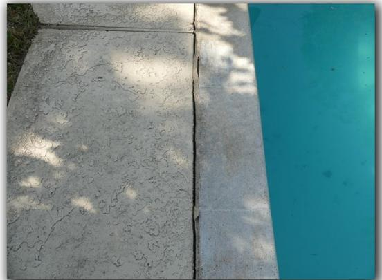
Pool/spa tiles, coping, and decks were observed to be cracked or damaged. The cause of cracked or damaged tiles, coping and decks should be determined and should be repaired or replaced as needed.
