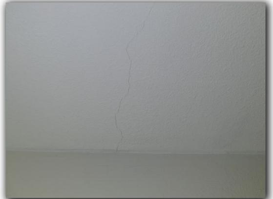
The ceiling drywall corner tape was observed to be pulling and twisting where walls and ceilings intersect. This condition is related to adverse foundation or structural performance and should be further evaluated by a certified, licensed foundation or structural specialist and repaired as needed.
