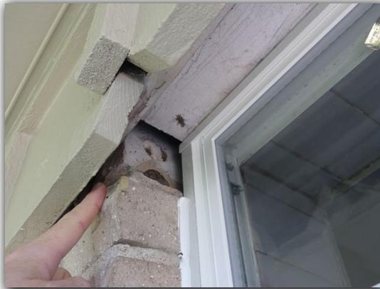
Peeling, damaged or deteriorating paint, stain and/or sealant was observed at the exterior wall cladding. Peeling, damaged and deteriorating paint or sealant should be repaired to prevent moisture penetration and deterioration of materials.
