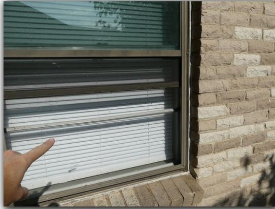
The windows need sealant between the window frames and exterior wall cladding. Lack of, damaged or deteriorating sealant around window frames may allow moisture and insect penetration and should be repaired as needed.
