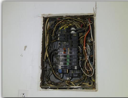
The electric service panel breaker use was not labeled. Each electric service panel breaker should be adequately labeled as to what appliance or circuit it serves.
