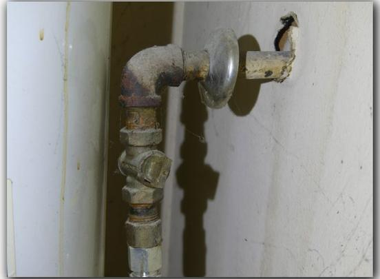
The gas supply flex connector at the heating equipment was observed to be passing through the heating equipment cabinet. Only rigid black gas pipe is allowed to pass through the heating equipment cabinet (appliance wall) (SAFETY HAZARD).
