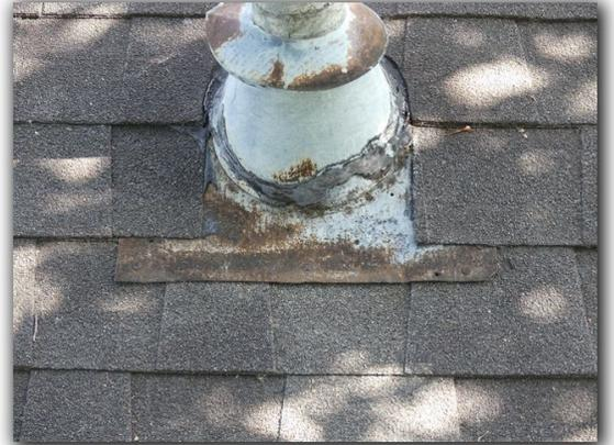
Roof covering flashings were observed to be lifting, damaged or improperly installed and were in need of repair or replacement. Lifting, damaged or improperly installed flashings may allow water penetration.
