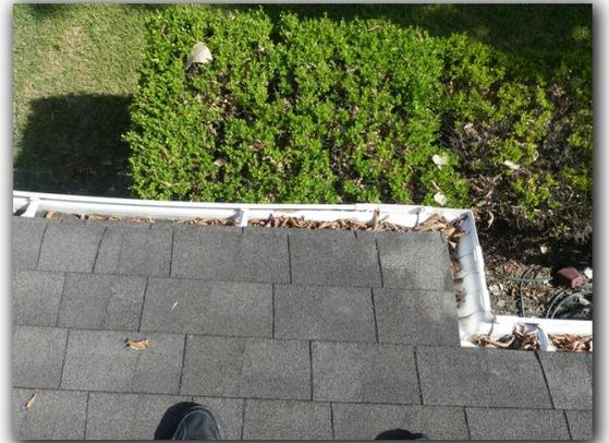
Planter(s) adjoining the structure create conducive conditions for wood destroying insects, moisture penetration and prevent the inspector from observing the foundation and or walls in these areas.
