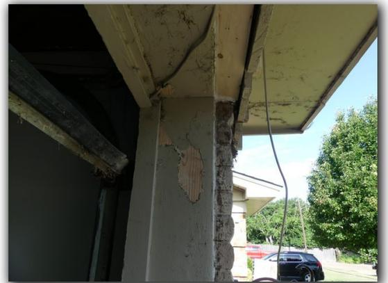
Some siding fasteners were observed to be not painted. Unpainted siding fasteners should be repaired.
