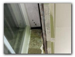
☑ Weep holes were not open, were missing and/or were improper spaced at the lower brick/stone of the exterior walls. Weep holes should be installed and properly spaced to provide proper wall ventilation.
