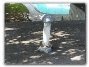
☑ The water heating equipment gas exhaust vent draft hood lacks screws that secure the draft hood to the flu. The draft hood and gas exhaust flu should be connected with screws to prevent separation. Separations between the draft hood and the gas exhaust flu are a SAFETY HAZARD and should be repaired prior to operation of the water heating equipment.
