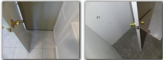
$\square$  Interior doors which are in contact with the floor covering should be repaired. Door which are in contact with floor covering may damage the flooring.
