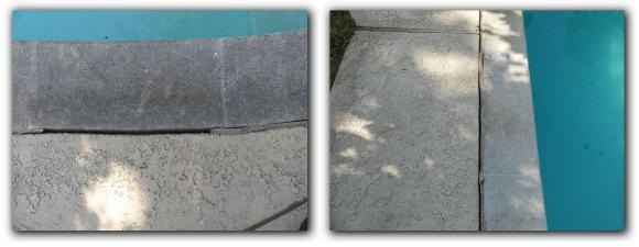
☑ Pool/spa tiles, coping, and decks were observed to be cracked or damaged. The cause of cracked or damaged tiles, coping and decks should be determined and should be repaired or replaced as needed.
