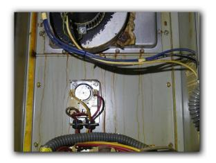
$\square$  Older style gas valves require a tool to operate at the heating equipment. Under current building standards, gas valves should be operable by hand.
