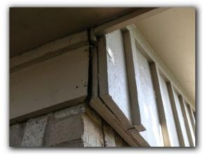
☑ Greater than normal separations between window frames and walls were observed which is an indication of movement, settlement or other defects that should be repaired. The cause of separations between walls and window frames should be determined and repaired as needed.
