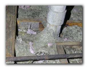
☑ The gas/flu vent has some portion that appears to be an asbestos material which is a known health risk and SAFETY HAZARD. Asbestos materials require specialized handling by a qualified specialist and should not be handled otherwise.
