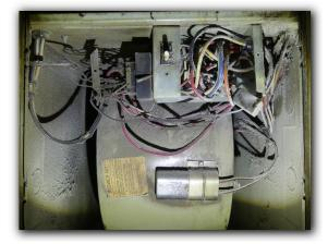
☑ The cooling equipment secondary condensation drain was not installed and did not have a secondary drain alarm or sensor installed. Current building standards state that all cooling equipment secondary condensation drain lines should drain to an observable location or have a water sensor/alarm installed in the secondary drain port.
