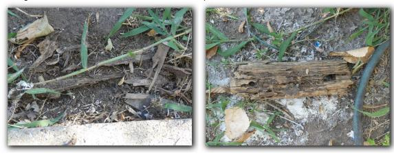
$\square$  Indications of **wood destroying insect damage or activity** was observed. There may be more damage than what was visible at the time if the inspection. Further evaluation is recommended.
