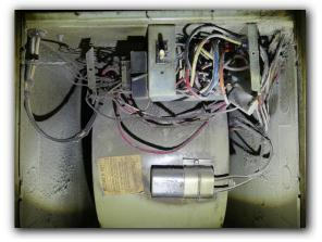
☑ Signs of rust or corrosion were observed at the heating equipment. Rust, corrosion or discoloration may be indications of age, wear, lack of maintenance or other defects. The heating equipment should be further evaluate by a certified, licensed heating equipment specialist and repaired or replaced as needed.
