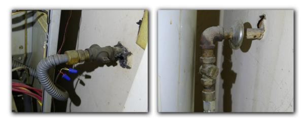
☑ The gas supply flex connector at the heating equipment was observed to be passing through the heating equipment cabinet. Only rigid black gas pipe is allowed to pass through the heating equipment cabinet (appliance wall) (SAFETY HAZARD).
