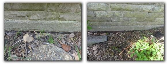
$\square$  Foundation slab corners have been sheared off (corner pop). This is a common condition in slab on grade foundations and should be repaired. Repairing corner pops is recommended to prevent moisture and wood destroying insect penetration.
