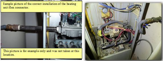
☑ There were gas fired appliances that did not have a "drip leg" installed. Under current construction standards, drip legs are required at the black iron gas pipe prior to a flexible gas line connection.
