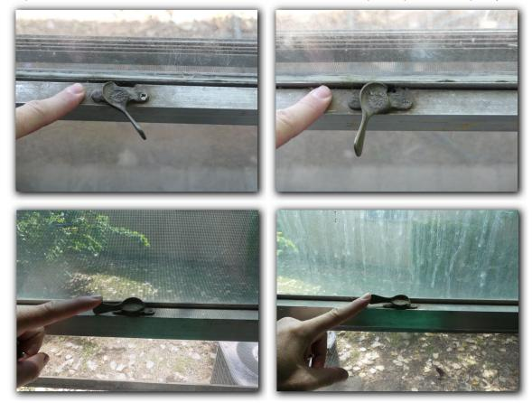
☑ Damaged window screens were observed. Window screens help protect window glass from minor impact damage and prevent insect penetration at the windows. Damaged window screens should be repaired or replaced.
