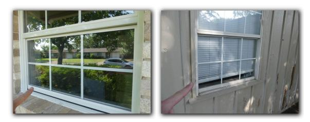
☑ The window above the tub/shower did not appear to have a safety glass etching or label. Glass less than 5' above the tub/shower should be tempered safety glass. Lack of safety glass in required locations is a SAFETY HAZARD and should be replaced.
