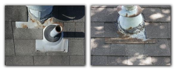
☑ Roof covering flashings were observed to be lifting, damaged or improperly installed and were in need of repair or replacement. Lifting, damaged or improperly installed flashings may allow water penetration.
