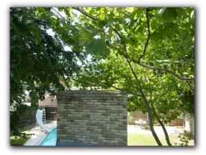
☑ The fireplace chimney lacks a metal cap. This condition should be further evaluated and corrected as necessary. Masonry chimney caps are often not visible and are known to crack which allows moisture to penetrate the structure. Masonry chimney caps are considered inadequate by current building standards and should be replaced with metal caps.
