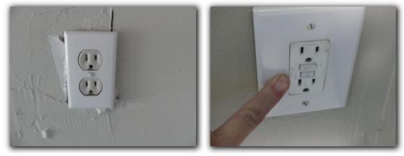
☑ Electrical receptacles, switches and or covers were observed to be loose, damaged, missing or missing screws and were in need of repair. Damaged or missing electrical receptacles or switches should be repaired by a certified, licensed electrical specialist.
