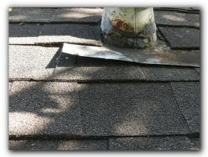
$\square$  Leave, sticks, branches and other debris were observed on the roof covering and may contribute to roof covering material damage and water penetration. The roof covering surfaces should be free of leaves, sticks, branches and debris.
