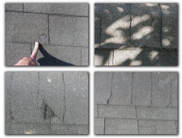
☑ Roof covering shingles that do not lay flat on the roof deck were observed. Roof covering shingles that do not lay flat on the roof deck were an indication of improper installation, damaged underlayment or other defects. Roof covering shingles that do not lay flat on the roof deck may allow further deterioration of the roof covering, deterioration of the roof structure, water penetration or other damage.
