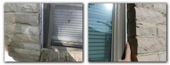
☑ The window weather-stripping was observed to be damaged. Damaged or missing weather stripping around windows may allow moisture penetration, conditioned air loss and insect penetration and should be repaired.
