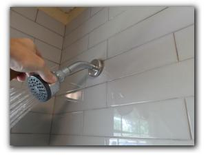
☑ The tub/shower water supply fixtures lacked adequate sealant at the wall. Tub/shower water supply fixtures should be properly sealed at the wall to prevent water damage.
