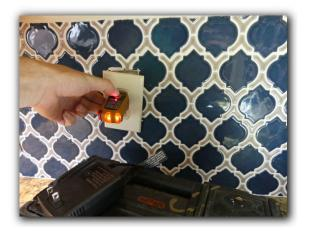
☑ The food waste disposer electrical receptacle was observed to lack ground fault circuit interrupter (GFCI) device protection. According to the 2014 NEC electrical standards, food waste disposer electrical receptacles should be GFCI protected. Lack of GFCI protection in required locations is a SAFETY HAZARD.
