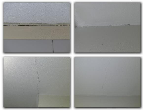
☑ The ceiling drywall corner tape was observed to be pulling and twisting where walls and ceilings intersect. This condition is related to adverse foundation or structural performance and should be further evaluated by a certified, licensed foundation or structural specialist and repaired as needed.
