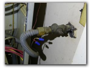
☑ The heating equipment gas exhaust flue was observed to be too close to combustible materials and was a SAFETY HAZARD. Defects in gas exhaust flues should be repaired prior to use of the equipment.
