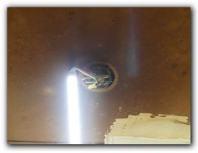
$\ensuremath{\boxtimes}$  Exterior light fixtures should be sealed at the wall to prevent water intrusion for reasons of SAFETY.
