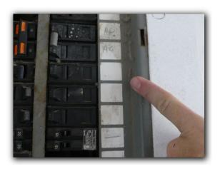
☑ The electric service panel cabinet cover plate or dead-front screws were observed to be sharp (SAFETY HAZARD) and should be replaced with the proper screws.
