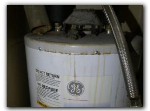
$\square$  The water heating equipment was installed without an overflow pan. Current building standards state that all water heaters should be equipped with an overflow pan with a drain that drains to the exterior of the structure if leaks would cause damage.
