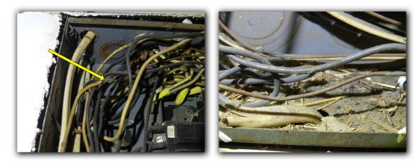
☑ Blank spaces (missing breakers) in the electrical service panel were observed to be missing filler covers. Missing or unused breaker slots should be covered with electrical fillers to prevent the unwanted entry of pests, moisture or other items. Lack of a cover filler at missing or unused breaker slots is considered a SAFETY HAZARD and should be repaired as needed by a qualified electrical specialist.
