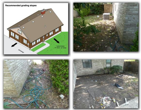
☑ High soil levels were observed at the foundation/brick line. 4 to 6 inches of the foundation perimeter beam should be visible. High soil levels may block weep holes and prevent proper wall ventilation. High soil levels create conducive conditions for wood destroying insects and water intrusion. High soil levels prevent the inspector from observing the foundation perimeter beam. Correction of inadequate grading clearance to exterior wall and foundation surfaces is recommended.
