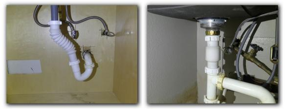
$\square$  Waste drains were slow to drain at sinks or tubs. The cause of slow drains should be determined and should be repaired or replaced as needed.
