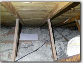
☑ Water stains were observed on the roof sheathing (decking). The cause of the water stains should be determined. You are strongly encouraged to have your insurance company and a certified, licensed roofing contractor to physically inspect the roof covering materials, prior to closing, to fully evaluate the insurability and condition of the roofing material.
