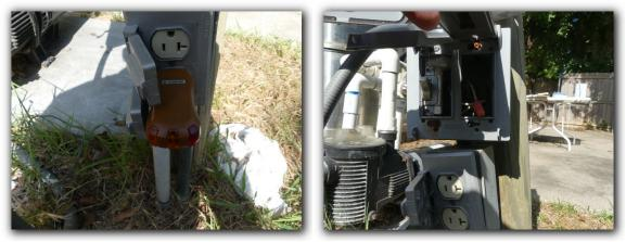
☑ Lack of bonding at pump motor, water heater, blower, or other electrical equipment to ground was observed to be a SAFETY HAZARD. Inadequate electrical bonding should be further evaluated by a qualified specialist.
