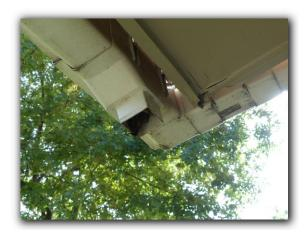
☑ The gutters and downspouts contained leaves and other debris and should be cleaned out to allow for proper drainage.
