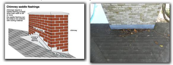
$\square$  The tree branches within 10' of the chimney were observed to be a SAFETY HAZARD and should be removed. Flammable materials such as tree limbs should not be within 10' of the chimney for reasons of safety.
