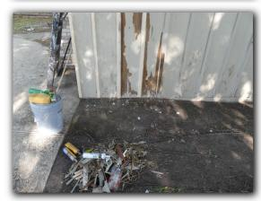
☑ Grading and drainage could be improved with the installation of rain gutters. Properly installed rain gutters can prevent erosion and water ponding and help direct water away from the foundation.
