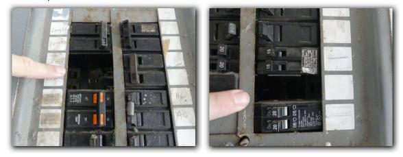
☑ Double tapped breakers were observed to be a SAFETY HAZARD in the electric service panel. Each breaker should provide electric service to only one circuit. The inspector recommends that the electric service panel be further evaluated and repaired or replaced as needed by a certified, licensed electrician.
