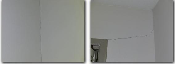
☑ Damaged or unfinished drywall was observed in the garage. Penetrations in ceiling or wall drywall between vehicle storage areas and living spaces are considered a SAFETY HAZARD and should be repaired.
