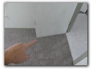
☑ Interior doors were observed to rub, stick or hit the door frames. Interior doors, that stick or hit the door frame may be an indication of movement, settlement or other defects. The cause of doors sticking or hitting door frames should be determined and repaired as needed.
