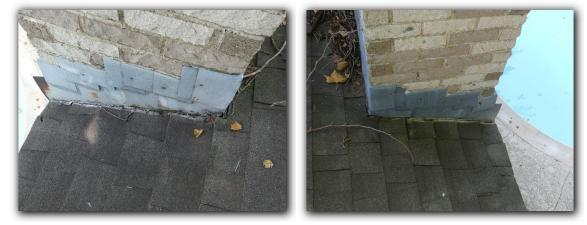
☑ Exposed nail heads were observed at the roof coverings. Exposed nail heads may allow water penetration and were in need of repair.
