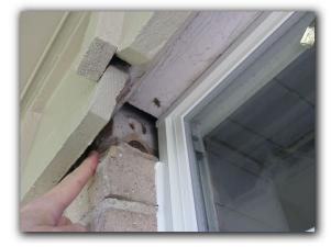
☑ Peeling, damaged or deteriorating paint, stain and/or sealant was observed at the exterior wall cladding. Peeling, damaged and deteriorating paint or sealant should be repaired to prevent moisture penetration and deterioration of materials.
