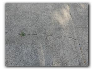
☑ Differential movement of the flatwork such as garage floors, driveways, walkways or patios was observed. Differential movement in flatwork may be an indication of movement, settlement or other defects and should be repaired as needed.
