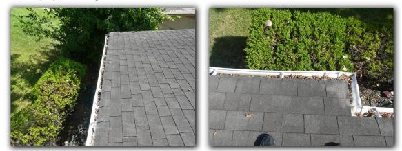
$\square$  Planter(s) adjoining the structure create conducive conditions for wood destroying insects, moisture penetration and prevent the inspector from observing the foundation and or walls in these areas.
