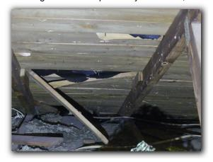
$\square$  Openings were observed in the attic at electrical, plumbing, duct work or other penetrations where they pass through structural framing. These opening should be sealed for improved FIRE SAFETY.
