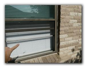
☑ The windows need sealant between the window frames and exterior wall cladding. Lack of, damaged or deteriorating sealant around window frames may allow moisture and insect penetration and should be repaired as needed.
