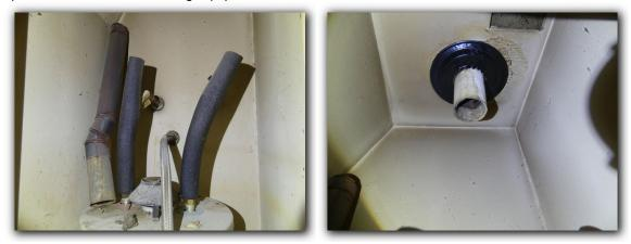
☑ The gas-fired water heating equipment was not properly vented for combustion and dilution air. Improper ventilation at the gas water heating equipment was observed to be a SAFETY HAZARD and may allow unwanted vapors to accumulate. Improper gas water heater ventilation may affect water heater performance. Further evaluation is recommended.
