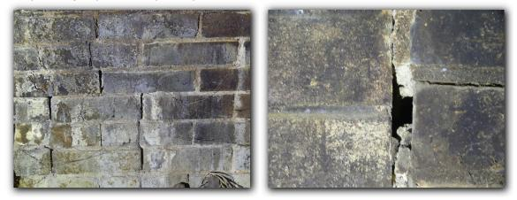
☑ The fireplace firebox brick/mortar was not sealed at the hearth or lintel and was a SAFETY HAZARD. Inadequate fireplace seals may allow heat to transfer to flammable materials and is a SAFETY HAZARD that should be repaired by a qualified fireplace specialist.
