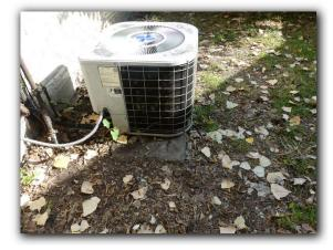
☑ The HVAC condenser unit coil fins were damaged / dirty and in need of service, repair or replacement. Dirty or damaged HVAC equipment coil fins may result in equipment damage, inadequate performance, reduced equipment life or other defects.
