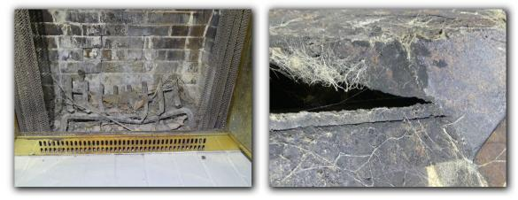
☑ The fireplace firebox brick and or brick mortar have been damaged. Damaged firebox brick or mortar may allow heat to transfer to flammable materials and is a SAFETY HAZARD that should be repaired by a qualified fireplace specialist.
