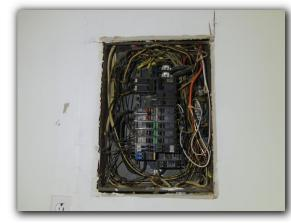
$\square$  The electric service panel breaker use was not labeled. Each electric service panel breaker should be adequately labeled as to what appliance or circuit it serves.
