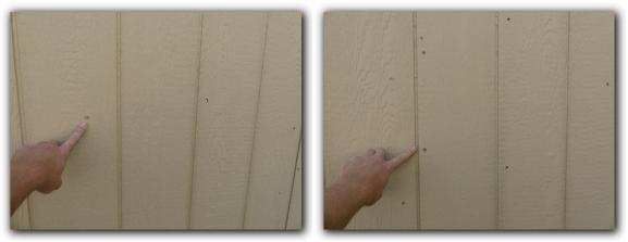
☑ Exterior sealants (caulking) were deteriorated or missing in some areas. Sealants applied in appropriate locations prevents moisture intrusion and insect penetration.
