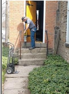
hammering the sunken and crooked concrete steps. Ultimately, the sacristy entry will have a small porch with railings and a timber frame roof. We're keeping an album of the progress and will post pictures along the way.
