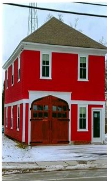
January 2024 photo of exterior renovation
