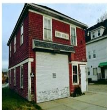
2011 photo of the station in disrepair
