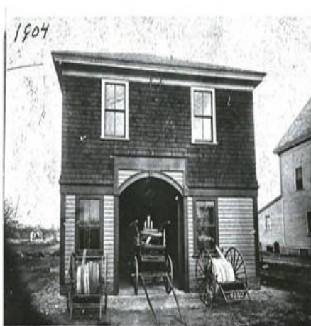
New North Uxbridge Fire Station built in the year 1904. Shown in photo are two hose reels and a horse drawn hand pumper. Note large door in center of station and no small side door.
