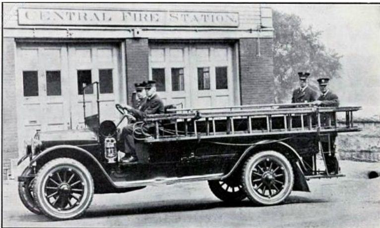
HOSE TRUCK BELONGING TO THE LITTLETON, N. H., FIRE DEPARTMENT
