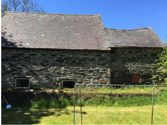
Building that houses the mill, mill pond in the foreground
