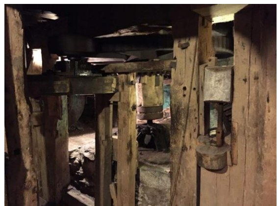
Basement of the mill
