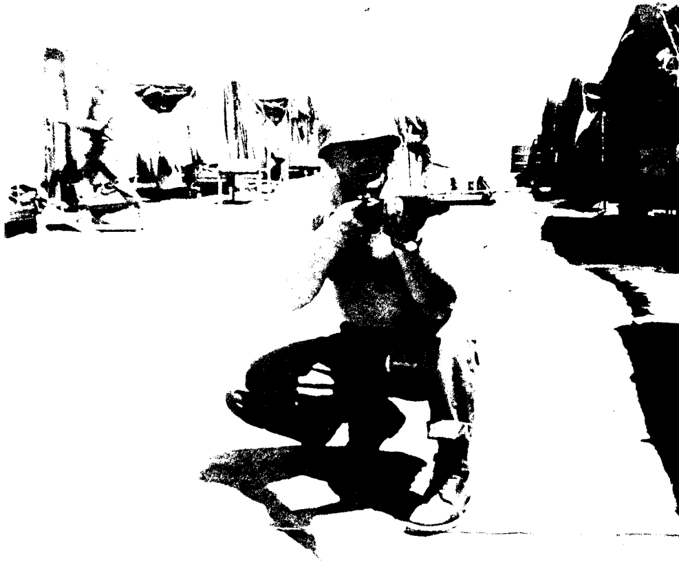
Don "Ike" Eminhizer at Seabee compound, CBD 1804 Det. Able, Korea. Summer 1952
