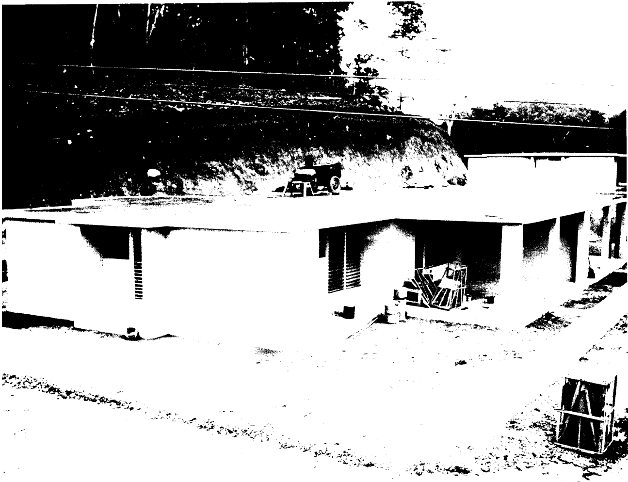
Haversack Housing – Close to completion
