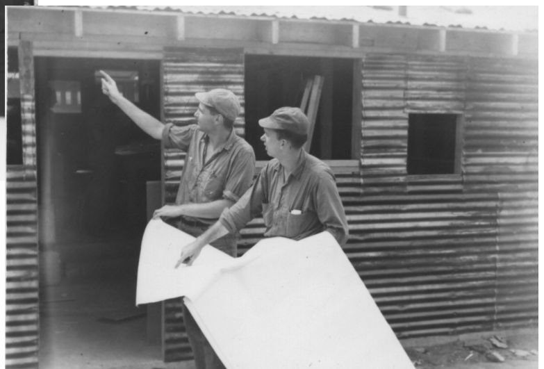
Right: Two brilliant engineers building highly secret building at undisclosed forward base in Korea. Petty Officer in Charge – Construction Crew #2: R.D. Thorp, BUL 2; Petty Officer in Charge – Engineering: H.V. Nelson, SV 2. (Yuk, yuk!)
