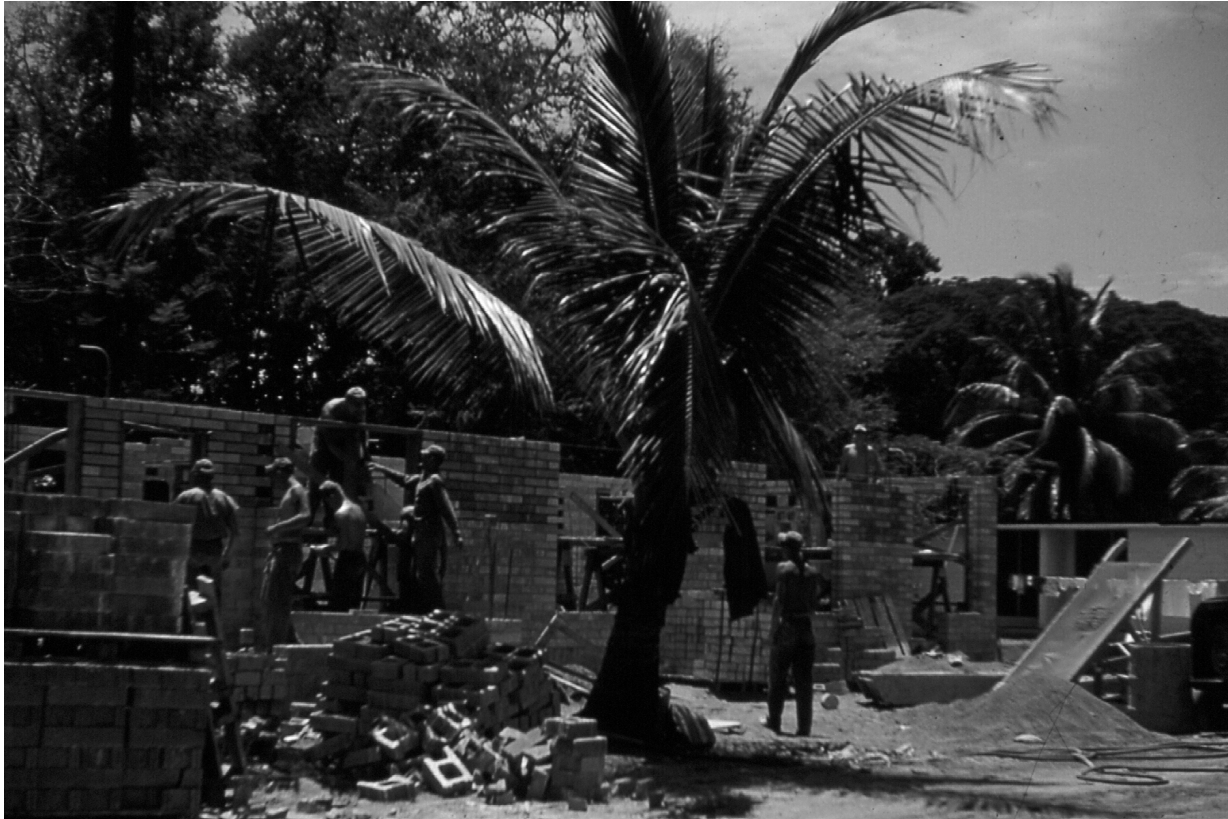
From 'Dutch' Klages. Sangley Point construction.
