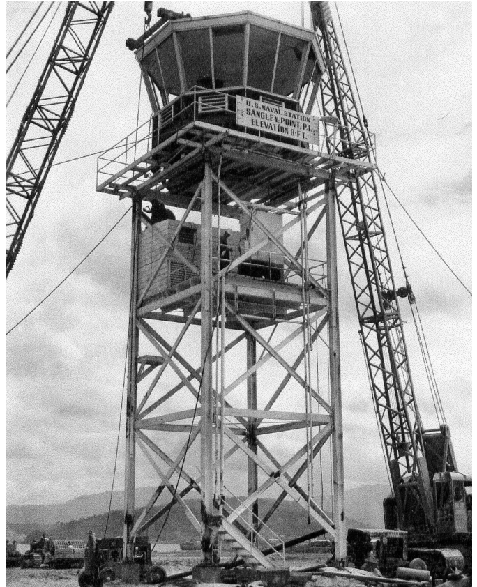
From Jack Foster: The control tower from Sangley Point being erected at Subic Bay. Jack is operating the crane on the left and Misner is operating the one on the right. Circa 1954.
