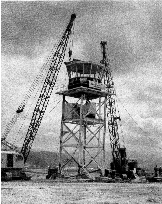
From Jack Foster: The control tower from Sangley Point being erected at Subic Bay. Jack is operating the crane on the left and Misner is operating the one on the right. Circa 1954.
