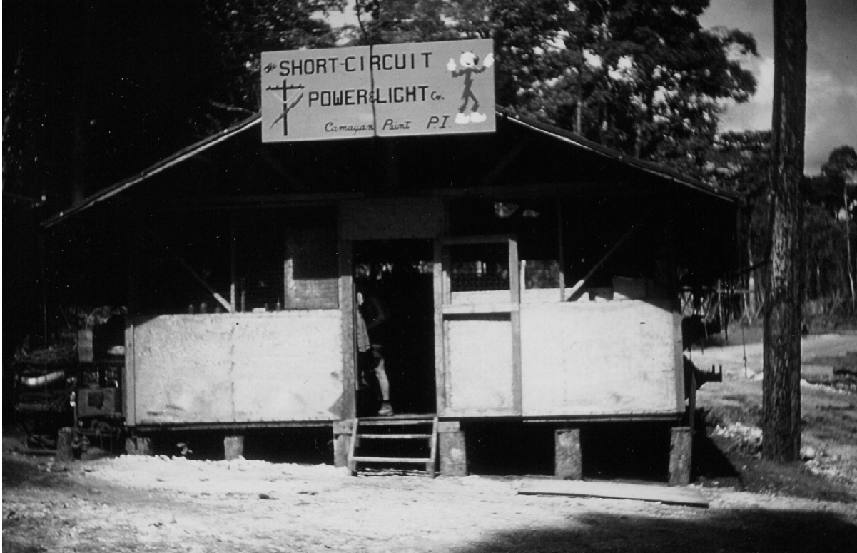
Above: The powerplant for Tent City, which had two generators that had to be synchronized each morning as they were rotated in service.
