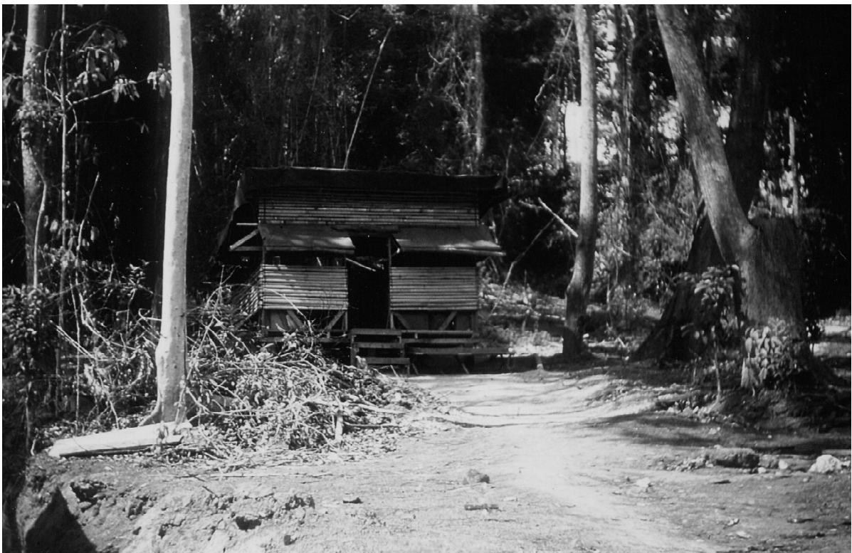
Above: The completed Clubhouse, with awnings and cured bamboo, September 1953.
