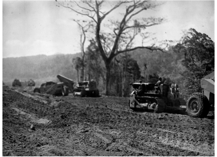
Building Camayan Road, Cubi Point, P.I., about 1952
