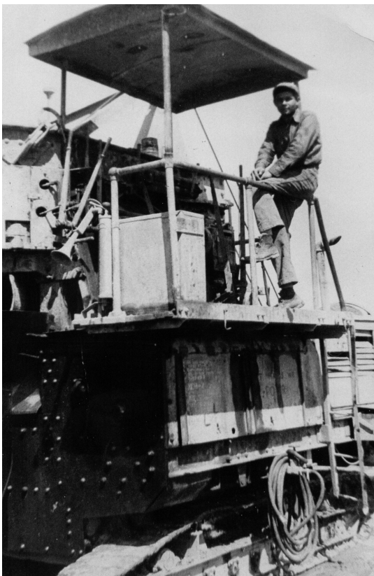
Ray Hooter operating the concrete paving machine, CBMU 1, K-3, Korea.
