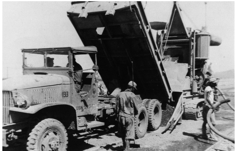
Runway paving crew, CBMU 1, K-3, Korea
