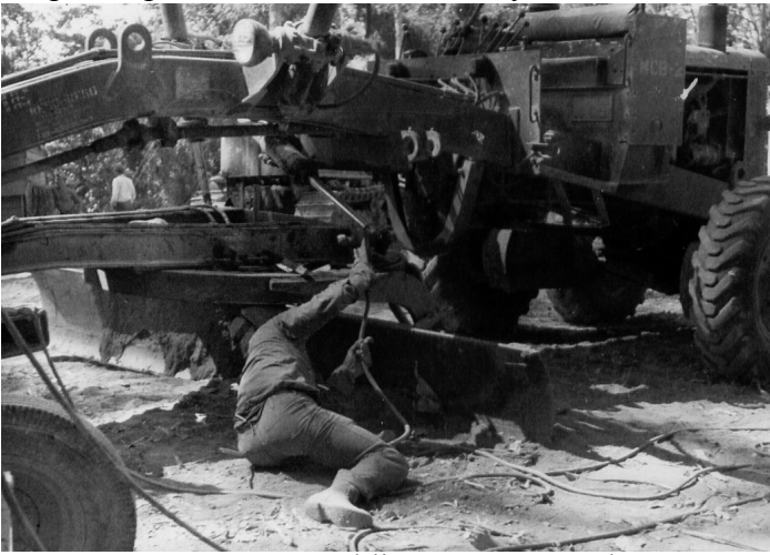
Sam Ragusa welding a motor grader, about 1952
