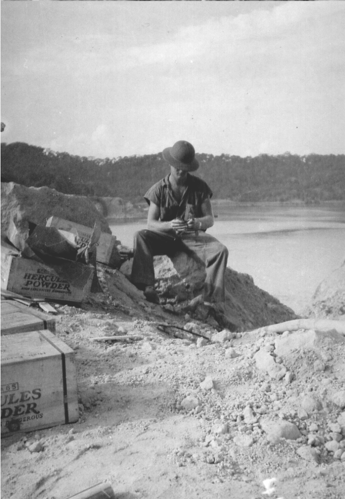
On top of the world! That's Cecil Westwood on top of Mt. Maritan preparing and setting the dynamite charges to bring Maritan down.
