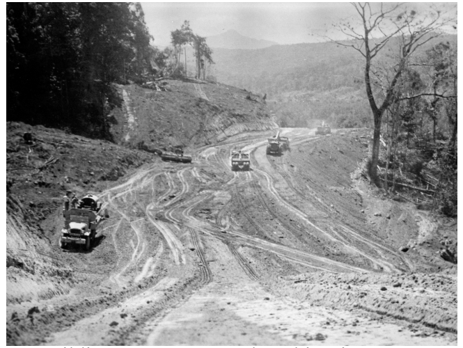
Building Camayan Road, Cubi Point, P.I., about 1952
