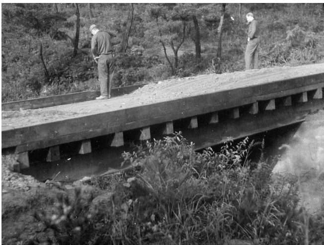
Karl Weisenbacher and William Ganske checking the bridge that was put up in a day. CBMU 1, Korea. 13
