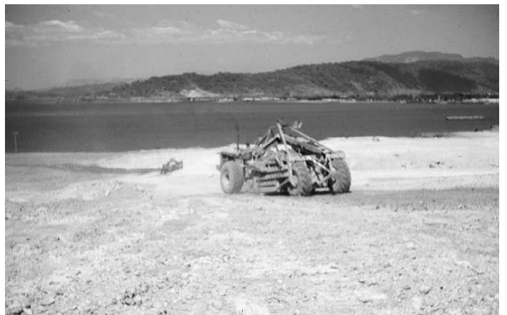
Building the runway at Subic Bay, ca 1954
