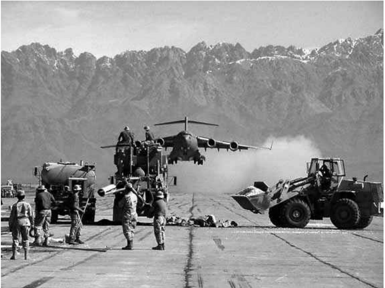
Seabees repairing a runway in Afghanistan—from Pat Morris
