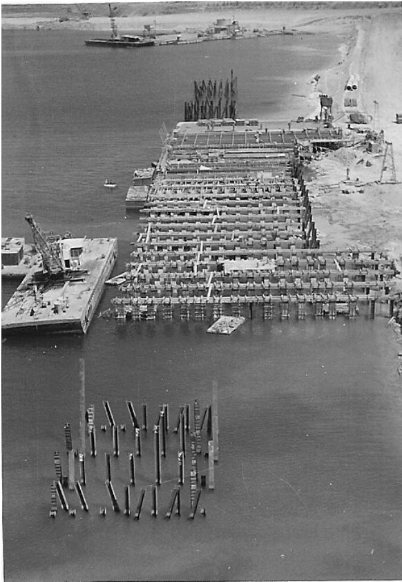
A couple of pictures at Subic Bay that are in my collection. The one of the cat that is turned over was taken at a road clearing site toward Camayan Pt. The other is of the carrier pier. I worked on a small raft putting concrete forms around the steel pilings. Once a month they had to send a diver down to pick up the dropped tools. The tool crib would run short on tools so this was a must. If a wooden-handle hammer was in the water for more than a month, the inside of the handle was honeycombed by the marine borers. LeRoy Weiselberg
