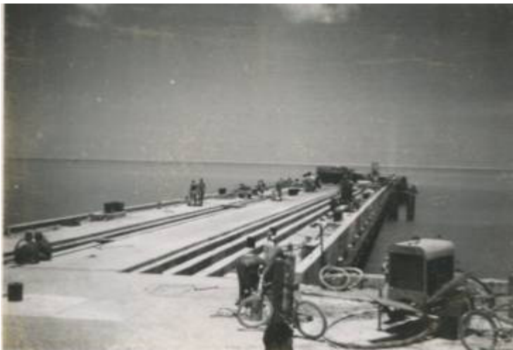
Pier No. 1 nearing completion. Built by MCB 2, Det. Able.
