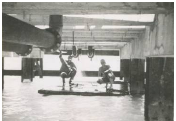
L-R: R.A. Guenther, UTCN; J.B. Bartman, UT 3. 16 Under Pier No. 1. 9 June, 1954
