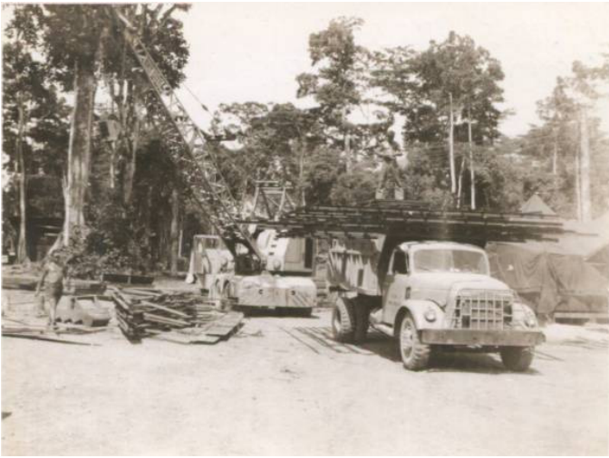
Above: Unloading structural steel, Camayan Point, June 1953.
