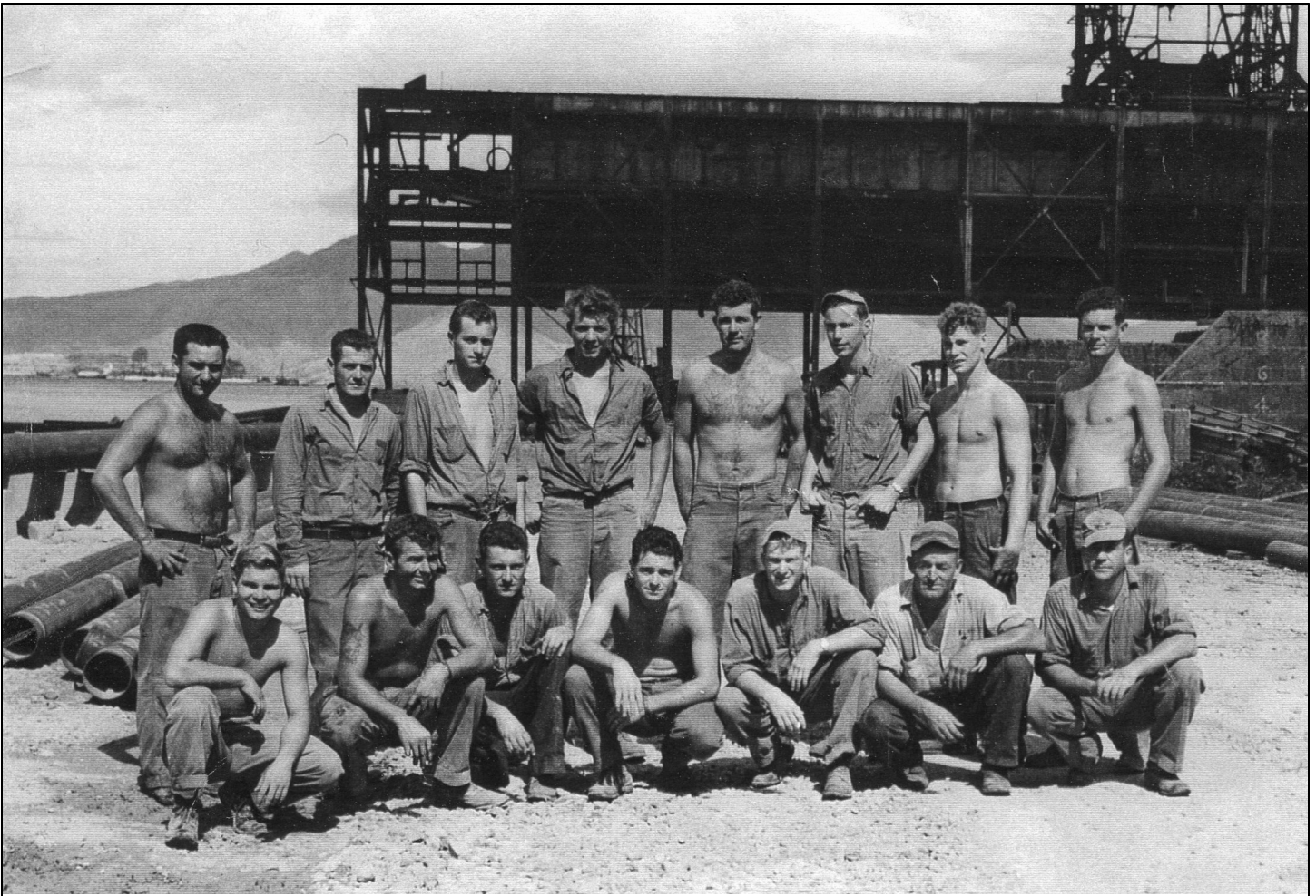
MCB 2 POL and Carrier Pier backfill crew, 1952, Cubi Point, Subic Bay, Philippine Islands. From Gene Robinson, third from left back row. Does anybody recognize these other men?
