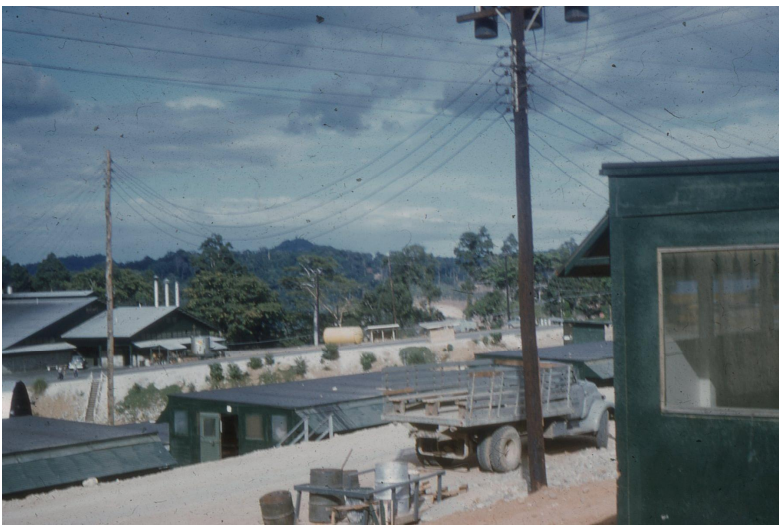
Overlooking Seabee camp area 1956.
