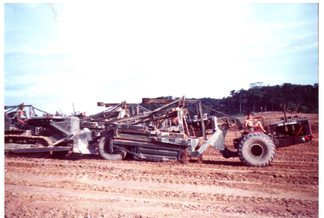
Cat and pan building airstrip - Cubi Point, Subic Bay, P.I.
