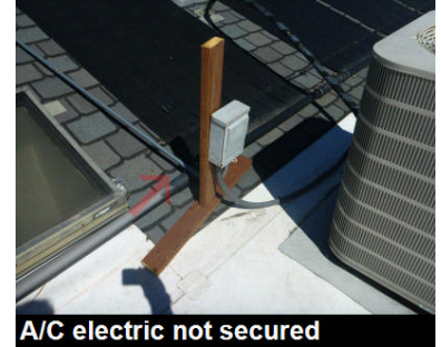
A/C electric not secured
