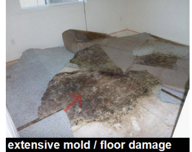
extensive mold / floor damage
