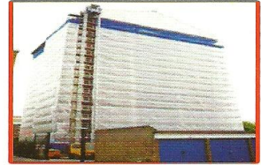
Scaffold Sheeting & Protection
