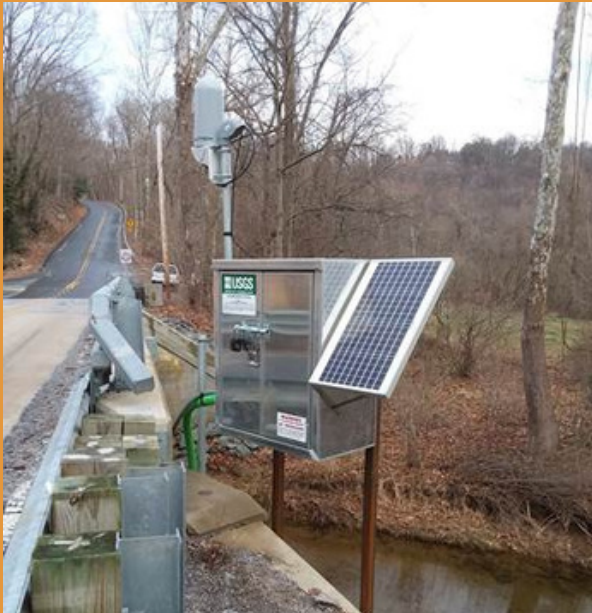
Monitor station at Fishing Creek, Craley.
