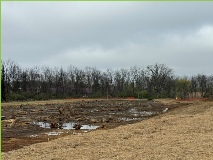
During construction in April.
