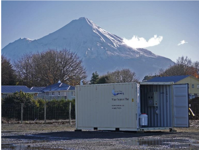
Rapid setup plants to provide urgent drinking water
