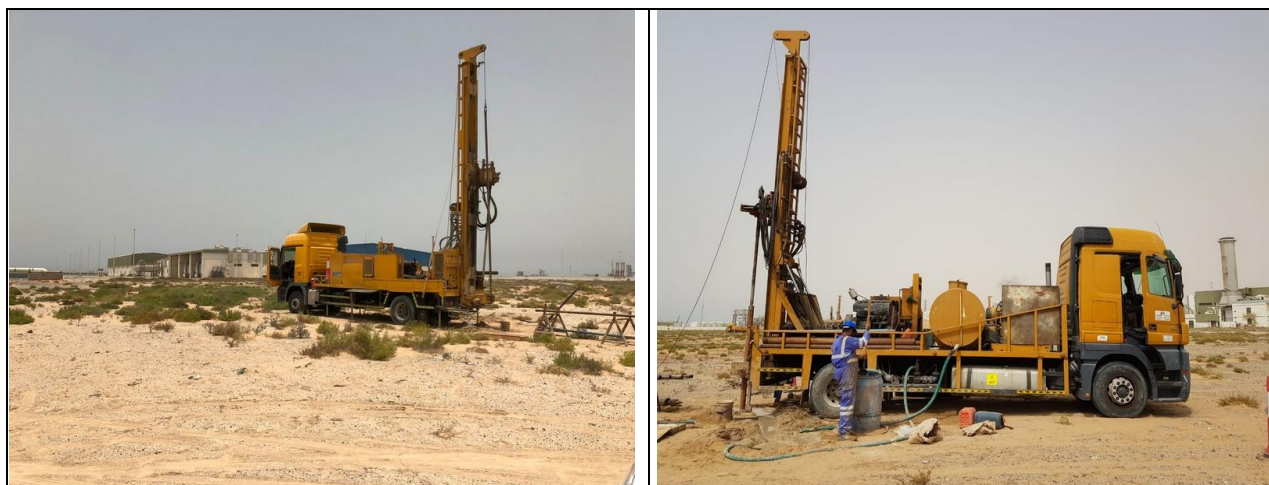
Figure 4: General photograph during drilling of boreholes
