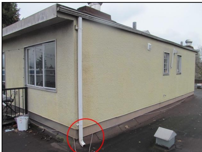
10. Discharge onto roofs
