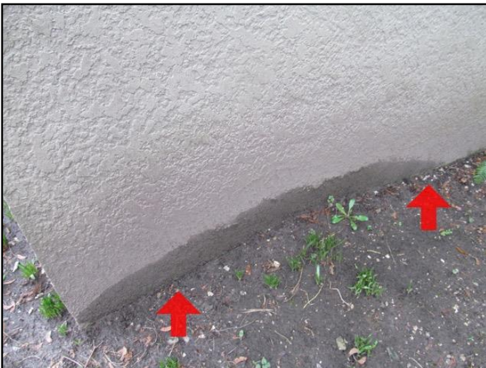
11. Too close to grade
