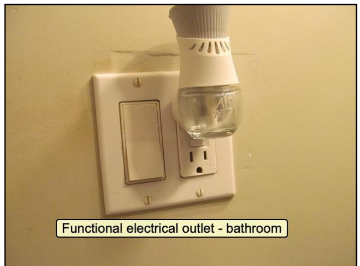
46. Functional electrical outlet - bathroom
