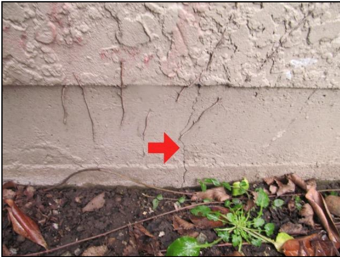
28. Typical minor cracks
