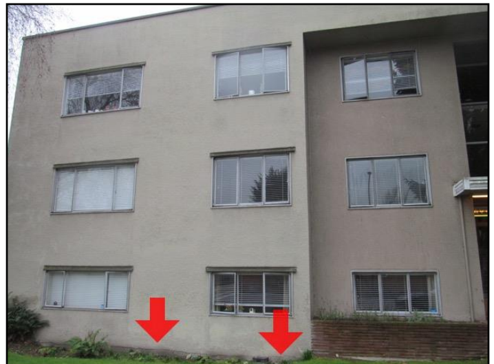
12. Too close to grade
