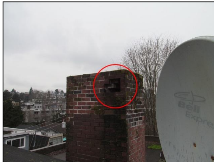
54. Loose, missing or deteriorated masonry
