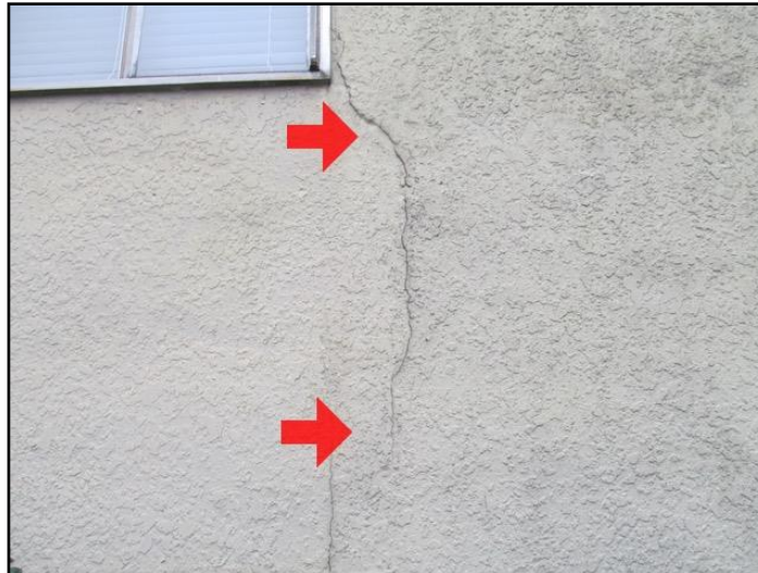
13. Minor cracks
