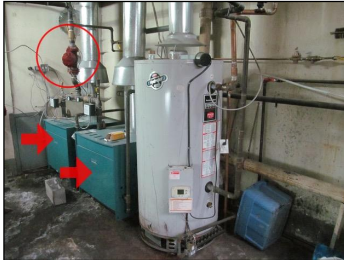
51. Gas hot water boilers
