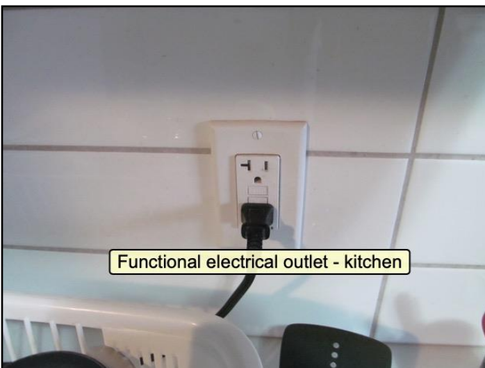
45. Functional electrical outlet - kitchen
