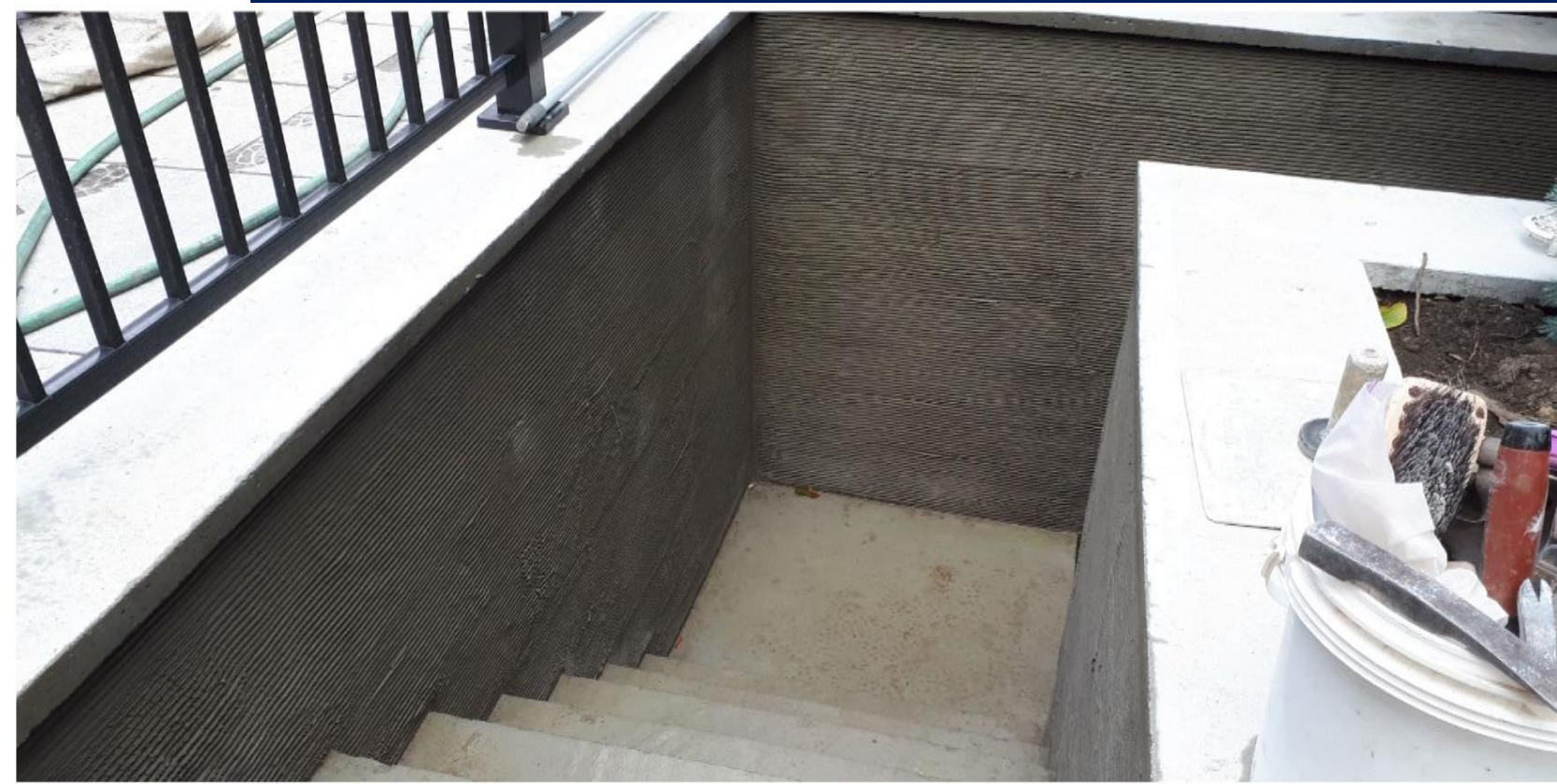
Picture above (before and after) Interior Plastering. Three coat application (base coat and veneer finish).
