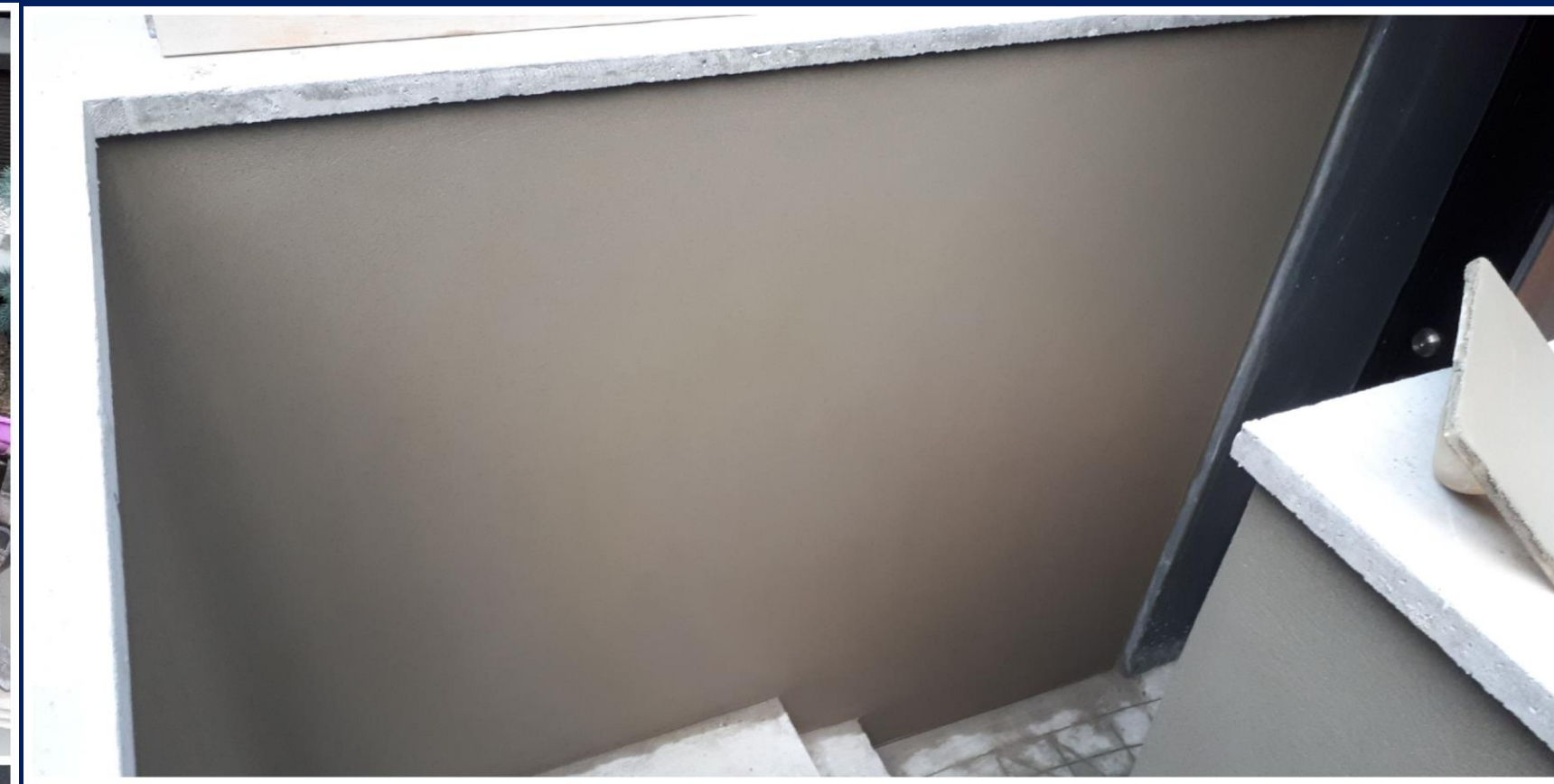
Picture above (before and after) Interior Plastering. Three coat application (base coat and veneer finish).
