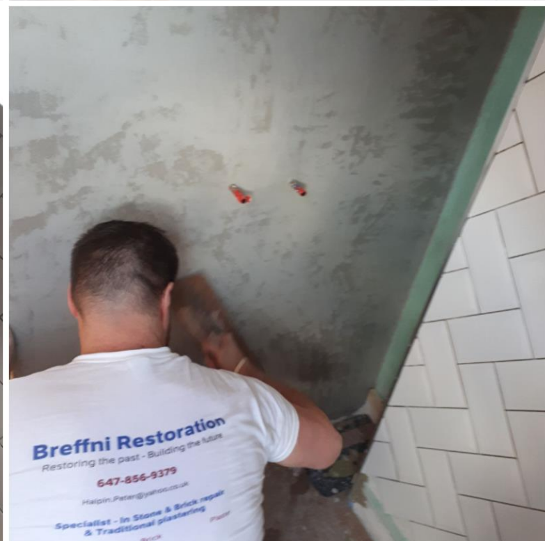
Picture above: Interior plastering with veneer finish Pictured to right (before and after): Float finish sand-cement plastering
