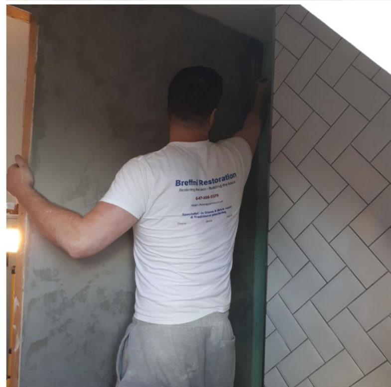
Picture above: Interior plastering with veneer finish Pictured to right (before and after): Float finish sand-cement plastering
