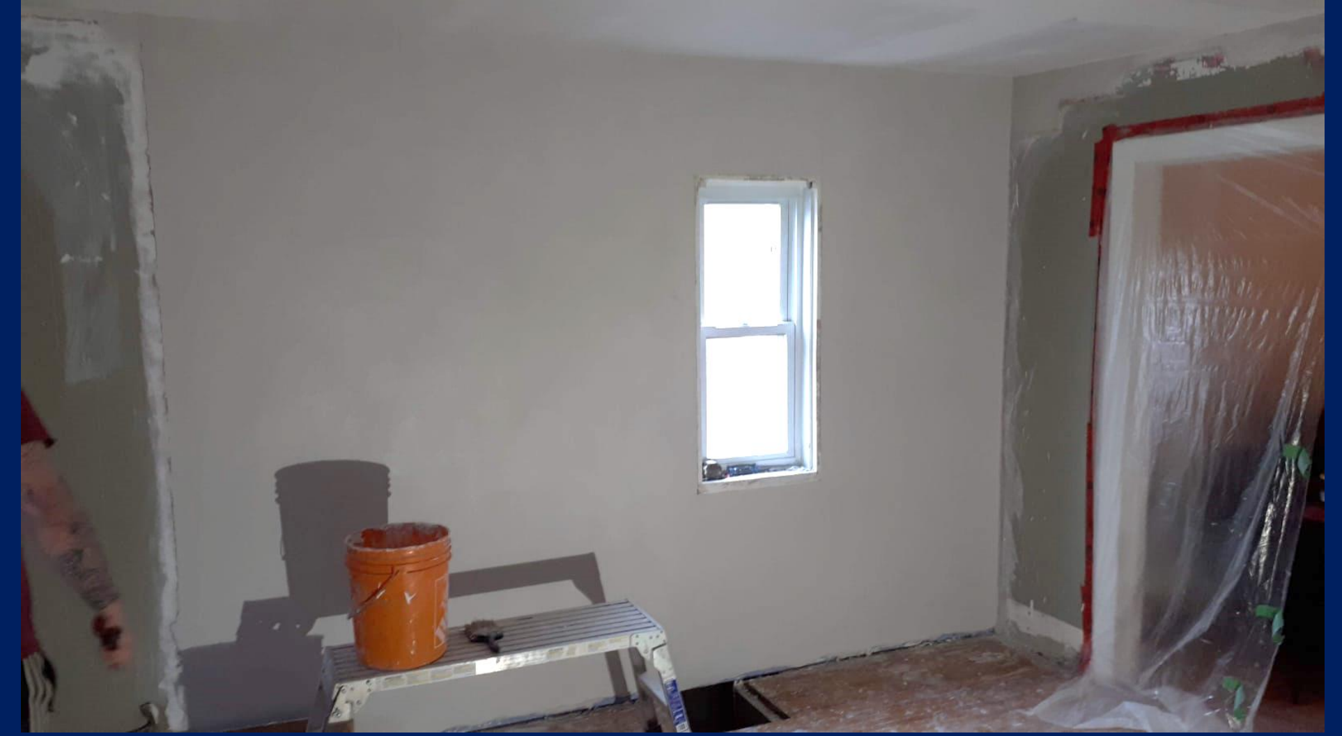
Picture above (before and after) Interior Plastering. Three coat application (base coat and veneer finish).
