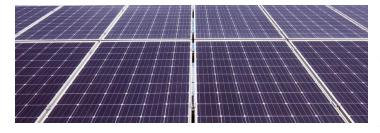
Solar panels convert sunlight into electricity through a process called the photovoltaic effect. During this process, solar panels collect electrons from the sun's light in the form of direct current (DC) electricity,
