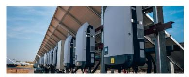
Inverters are the brains of a solar power system. They are responsible for converting DC power (from your panels) into AC power (the format that is usable by your household appliances). They also route the flow of electricity between system
