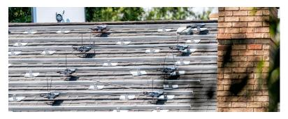
Racking is the foundational structure that secures your solar panels in place. Racking systems come with mounting rails and flashings to secure the rails to your rooftop or ground mount.
