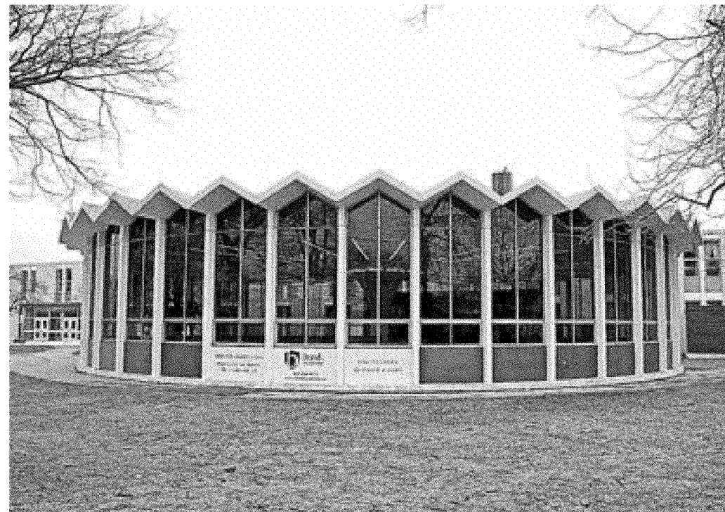
A single mushroom-shaped column holds a circular roof aloft to form a crown at the Bond Academy, a building constructed in 1961. DAVE LeBLANC
