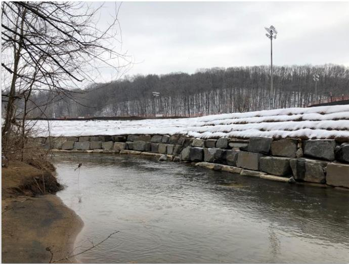
**Figure 5.** Geobag system after installation with added toe rock protection
