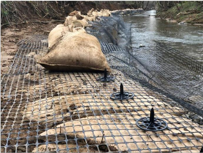
**Figure 4.** Geobag system installation
