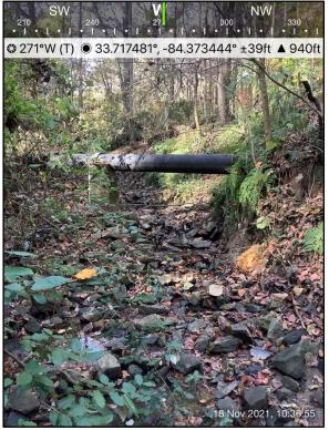
Photograph 15: Sanitary sewer crossing near confluence of Stream 1 and Stream 3 at approx. Sta. 5+00
