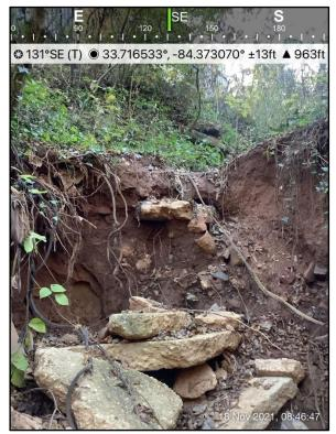
**Photograph 1**: Erosional drainage feature adjacent to abandoned culvert structure looking upstream along Stream 1
