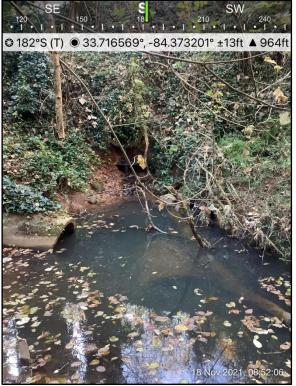
**Photograph 3**: Primary culvert structure draining to Stream 1 looking upstream at erosional plunge pool and relic culvert structure in the foreground
