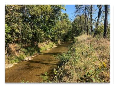
Figure 6. Geobag system fully stabilized and vegetated
