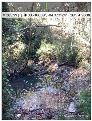
**Photograph 5**: Plunge pool feature from outlet of primary culvert drainage structure along Stream 1 looking downstream
