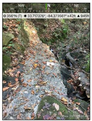
**Photograph 13**: Concrete pipe protection over sanitary sewer line at large headcut along Stream 1 at approx. Sta. 4+70
