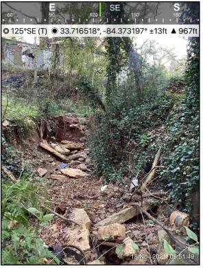
**Photograph 2**: Erosional drainage feature adjacent to abandoned culvert structure looking upstream along Stream 1
