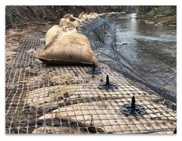
Figure 4. Geobag system installation
