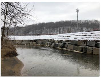
Figure 5. Geobag system after installation with added toe rock protection
