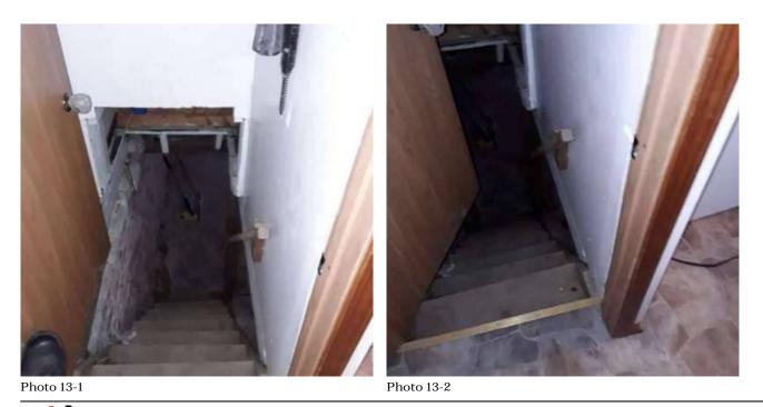
14) + Chandrails at one or more flights of stairs were too low or too high and pose a fall hazard. Handrails should be located at least 34 inches and at most 38 inches above the nose of each tread/riser. Recommend that a qualified person repair per standard building practices.
