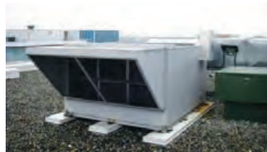
Typical rooftop make-up air unit
