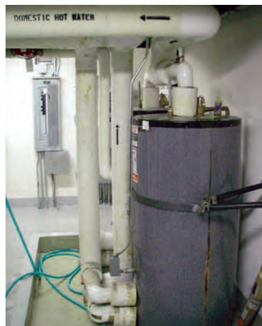
Central domestic hot water system
