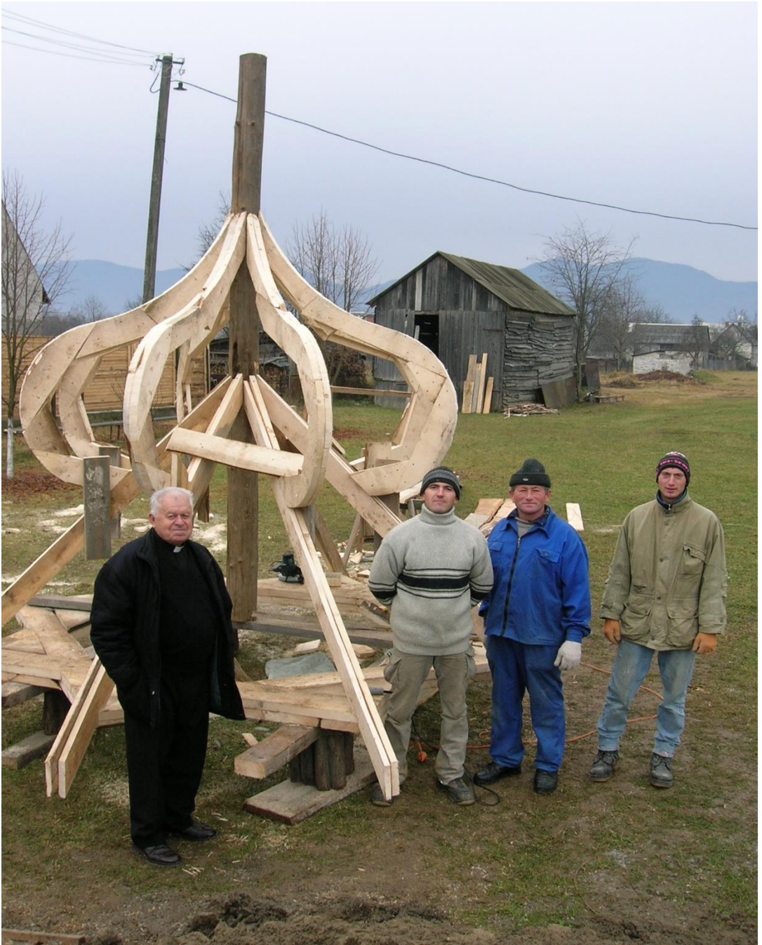
Fr. Stephan Cych supervises church construction near Khust in Zakarpatya
