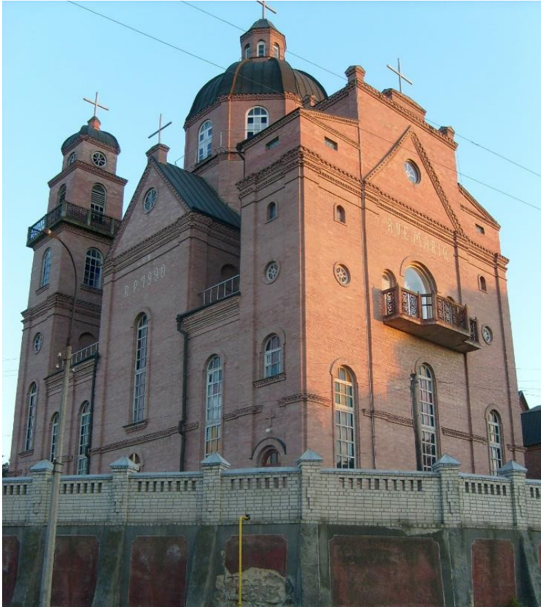
QAMA supported monastery construction in Novograd-Volinsky.
