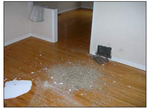
Vermiculite insulation spilled from an attic during a renovation
