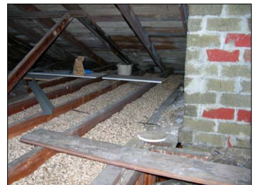
Typical vermiculite insulation in an attic
