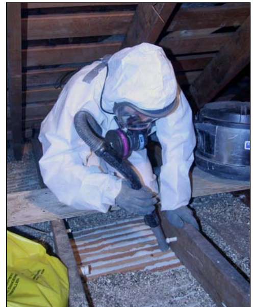
Protected asbestos worker removing vermiculite insulation from an attic
