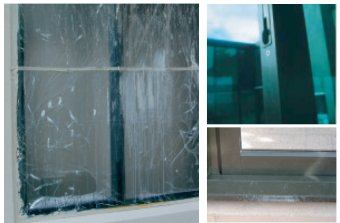
Three of these photographs display damage that has occurred on site, post installation. The photo of the masked joinery on the left displays clear signs of damage that could have occurred were it not masked. Please ensure that your joinery is protected right through the entire construction process.
