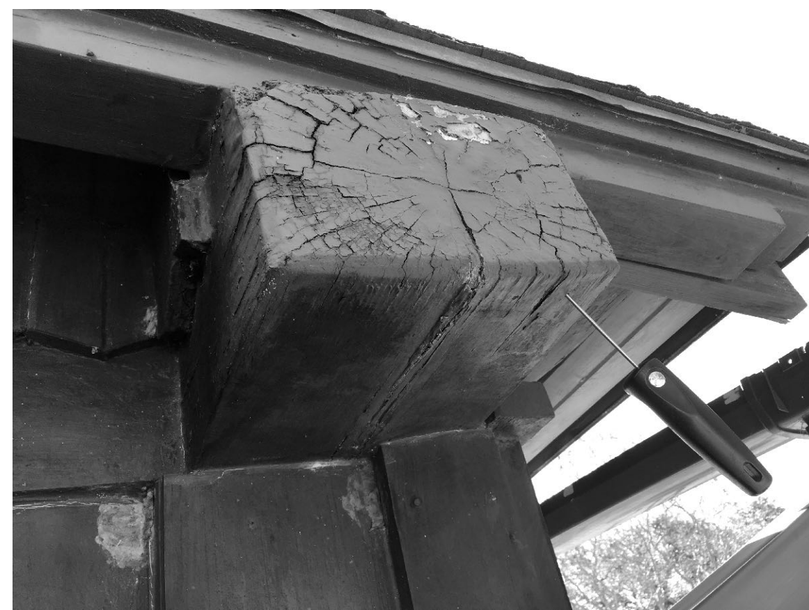
PHOTO 5 EAVE AT SOUTH ENTRY
