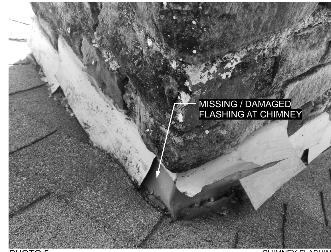
PHOTO 5 CHIMNEY FLASHING
