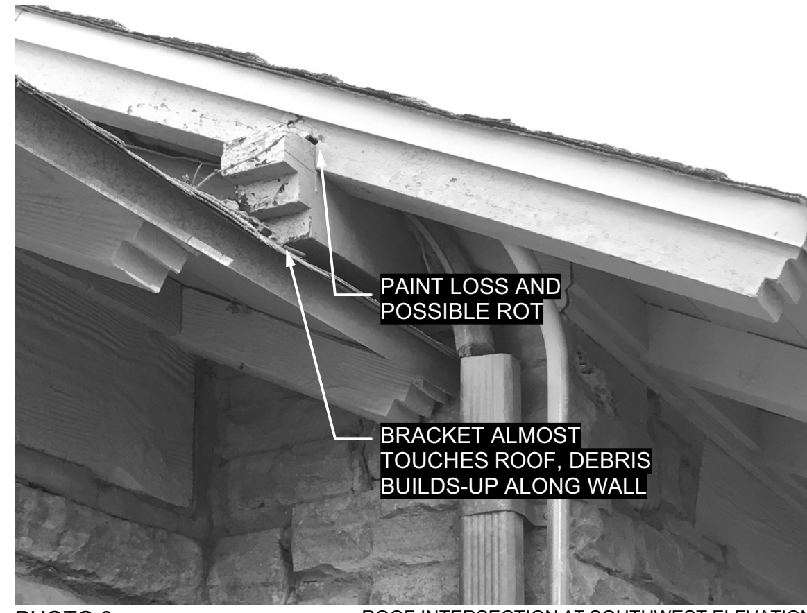
PHOTO 6 ROOF INTERSECTION AT SOUTHWEST ELEVATION
