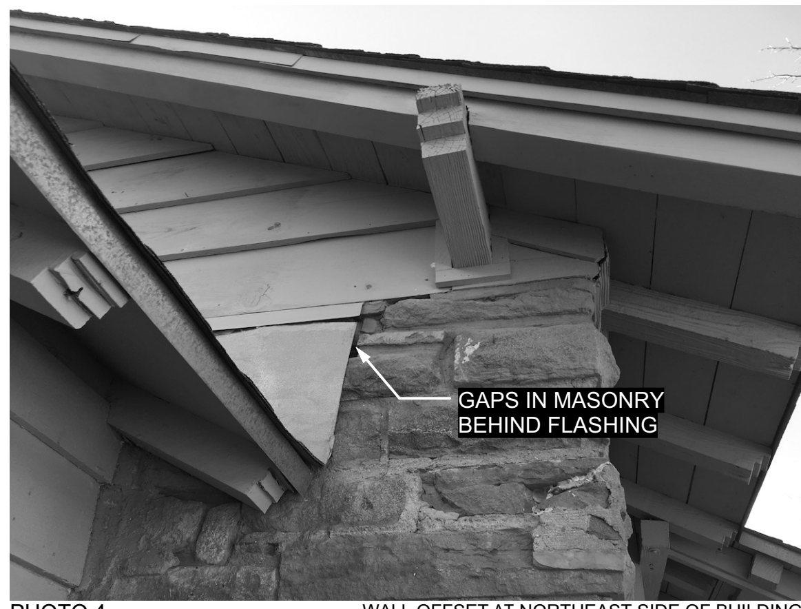
PHOTO 4 WALL OFFSET AT NORTHEAST SIDE OF BUILDING
