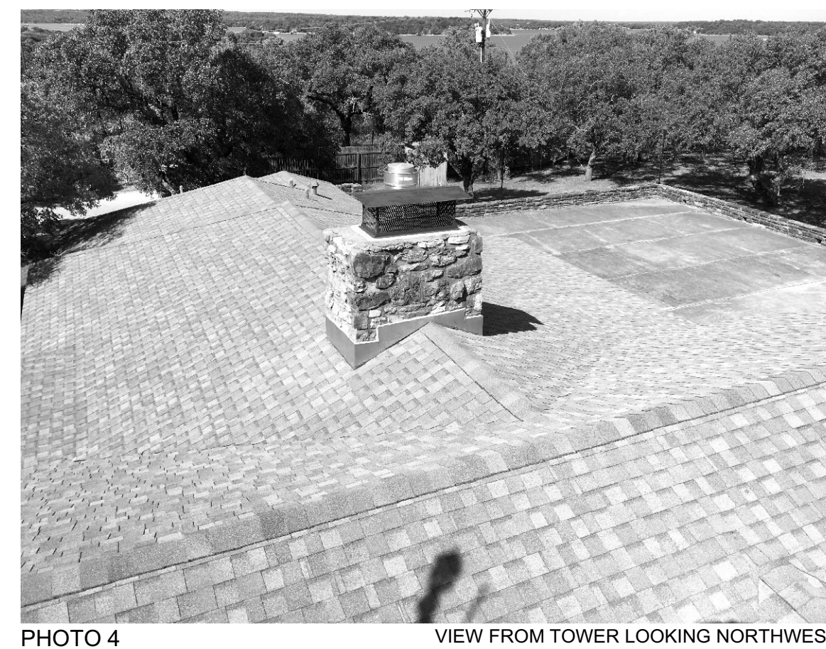
PHOTO 4 VIEW FROM TOWER LOOKING NORTHWEST
