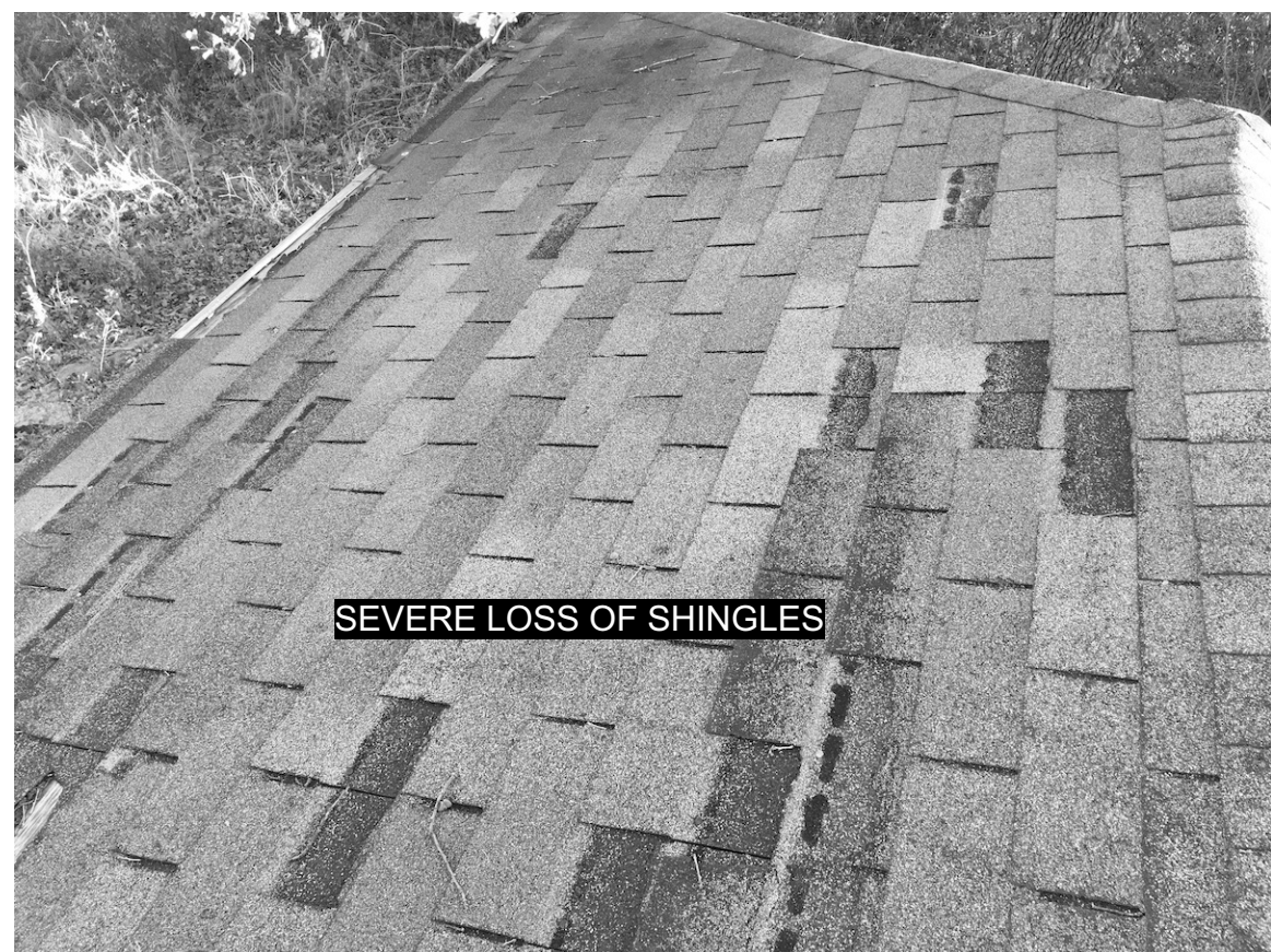
PHOTO 7 SEVERE LOSS OF SHINGLES ROOF LOOKING SOUTH
