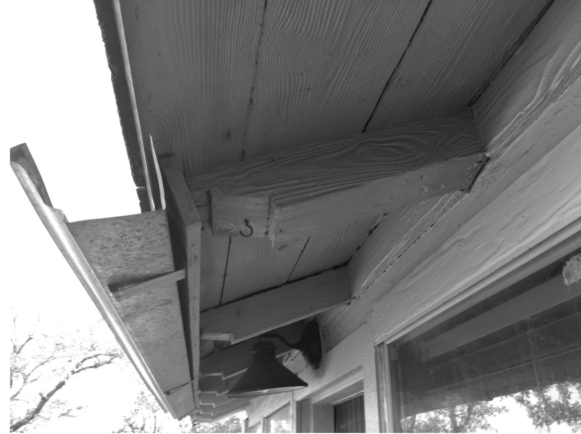
PHOTO 4 EAVE AND GUTTER AT SOUTHEAST
