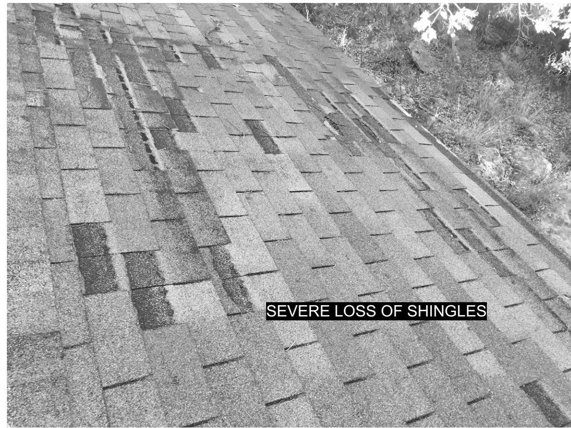
PHOTO 6 SEVERE LOSS OF SHINGLES ROOF LOOKING NORTH
