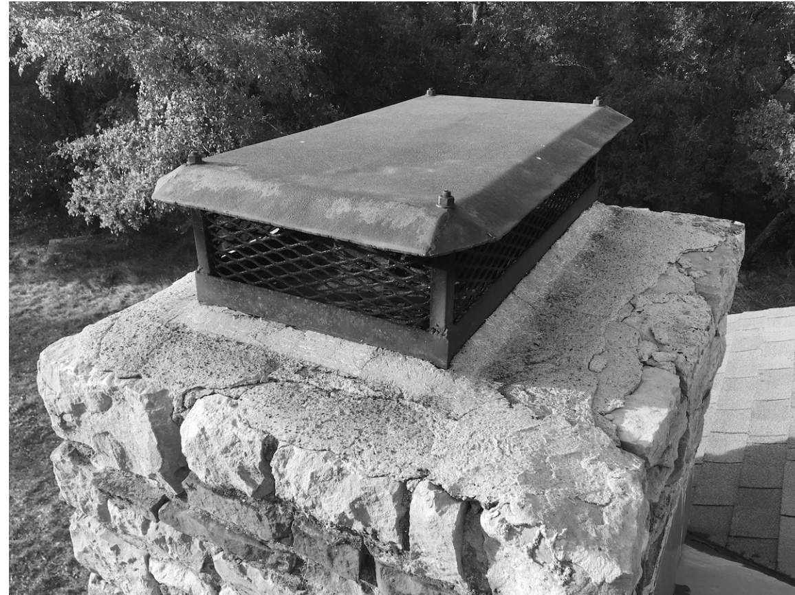
PHOTO 7 DETAIL AT CHIMNEY CAP
