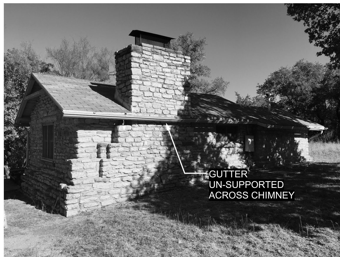
PHOTO 1 VIEW FROM NORTHWEST
