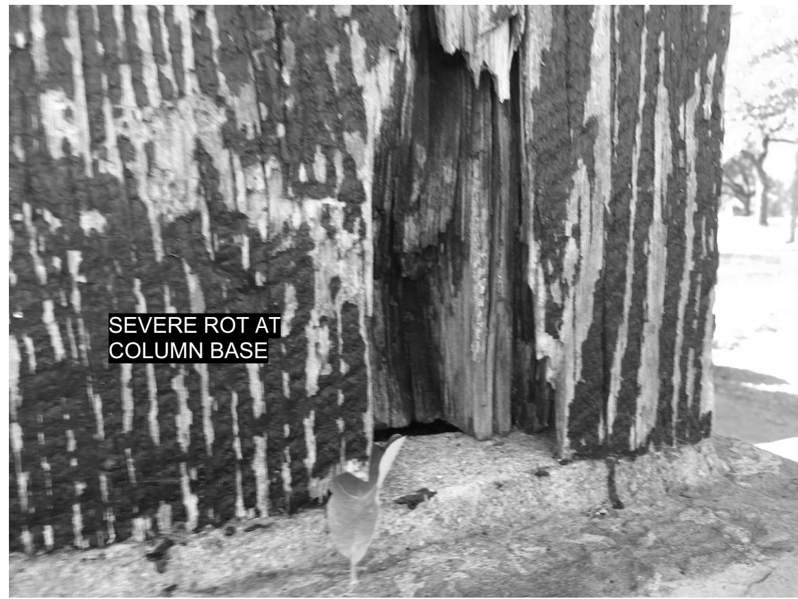
PHOTO 3 SEVERE ROT AT COLUMN BASE
