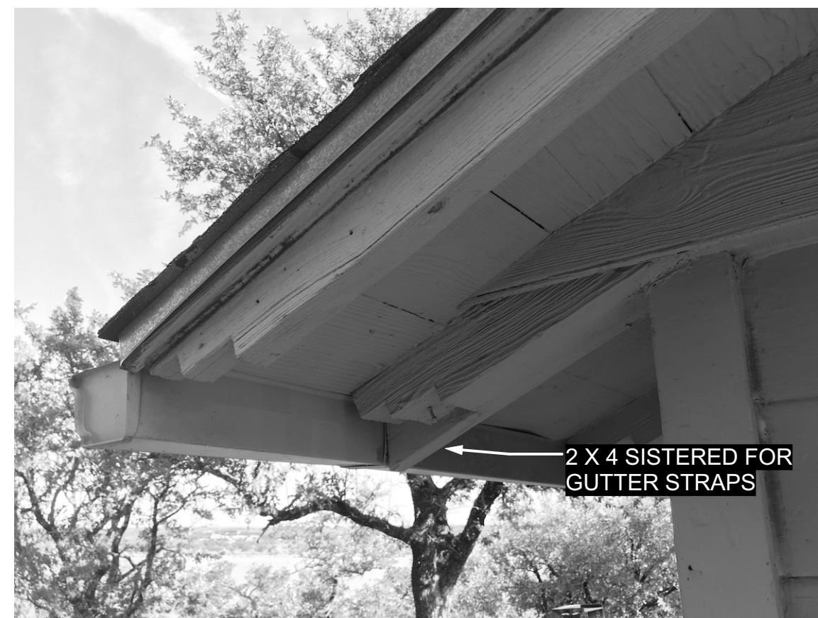
PHOTO 8 EAVE AT WEST ELEVATION
