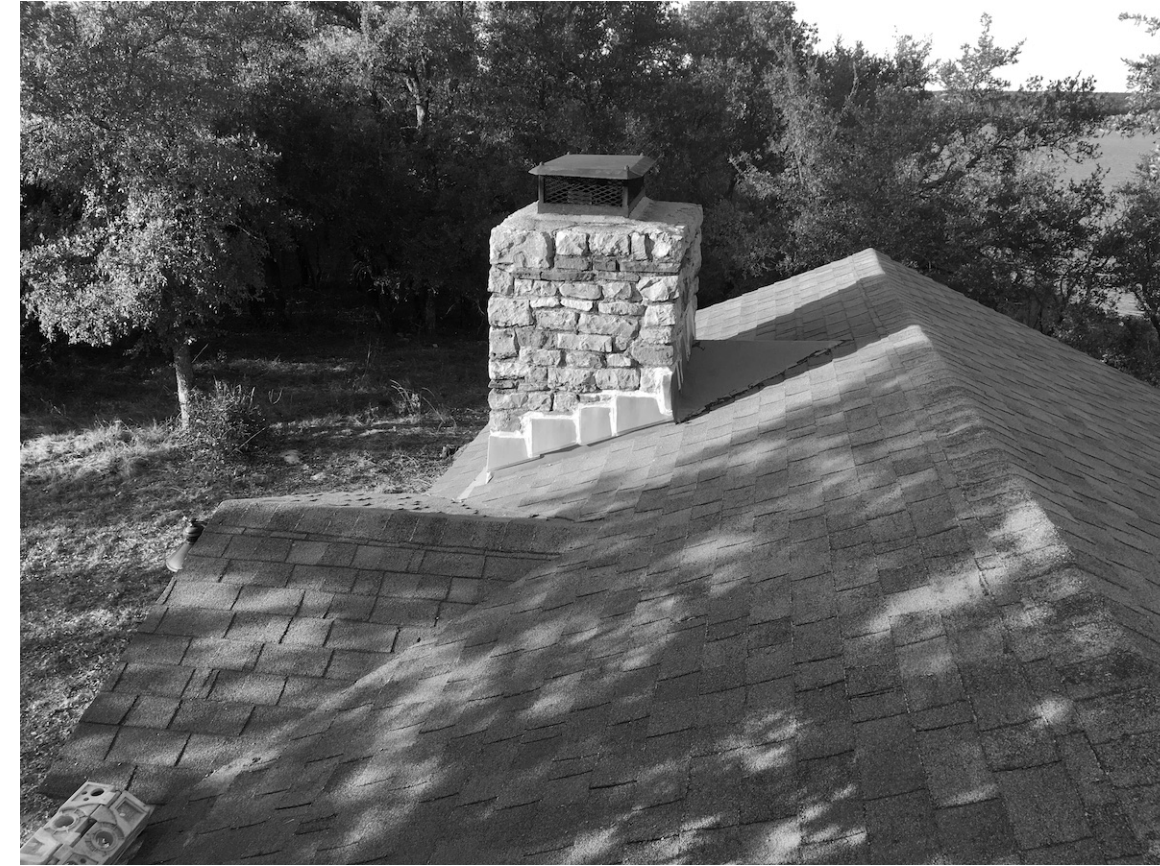
PHOTO 6 ROOF LOOKING NORTH
