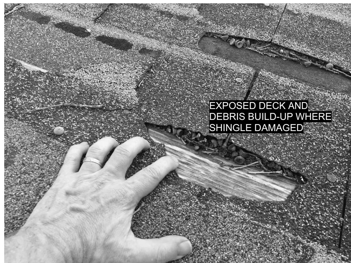
PHOTO 8 EXPOSED DECK AND DEBRIS BUILD-UP WHERE SHINGLE DAMAGED
