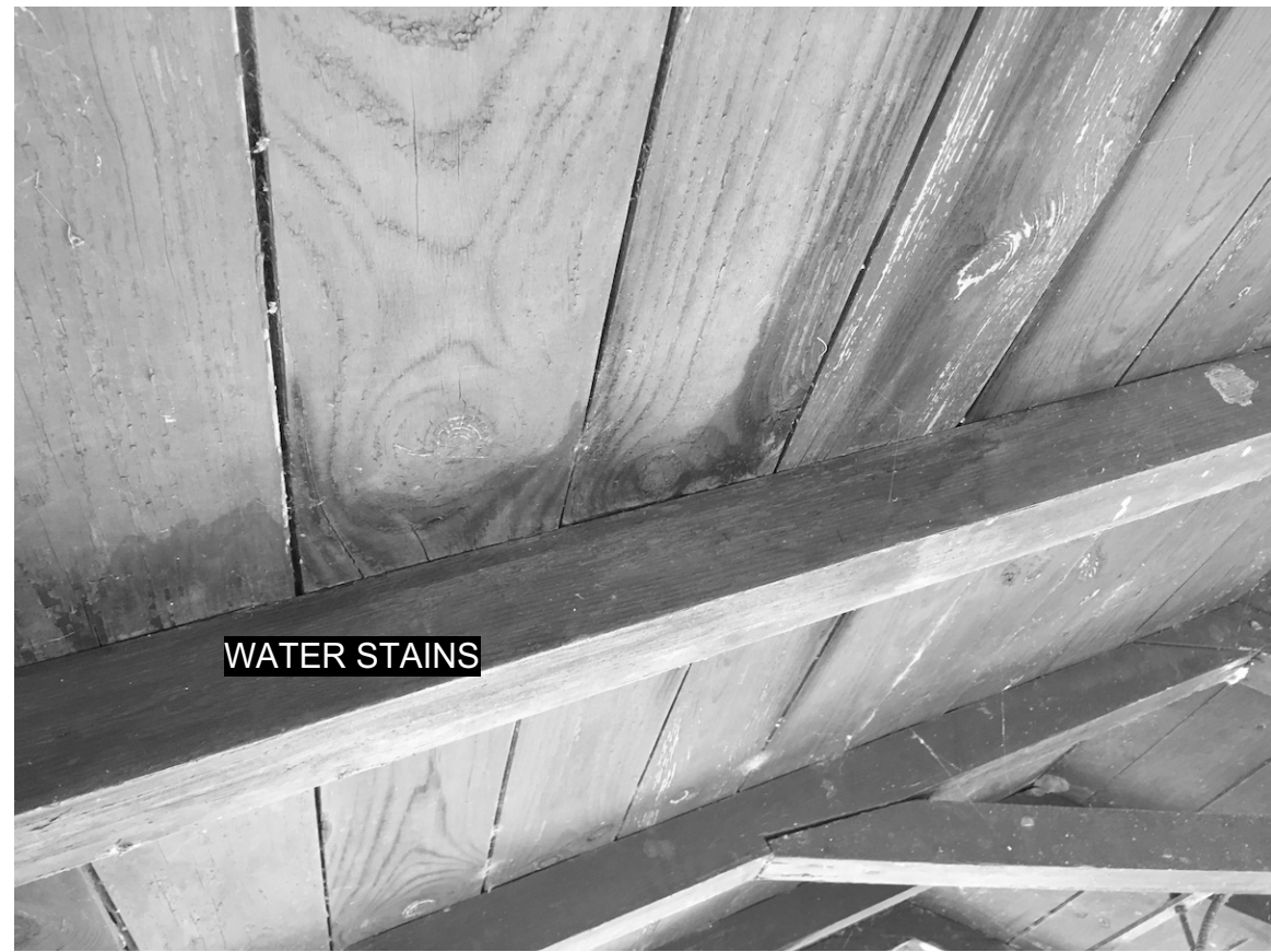
PHOTO 5 WATER STAINS AT DECK UNDERSIDE
