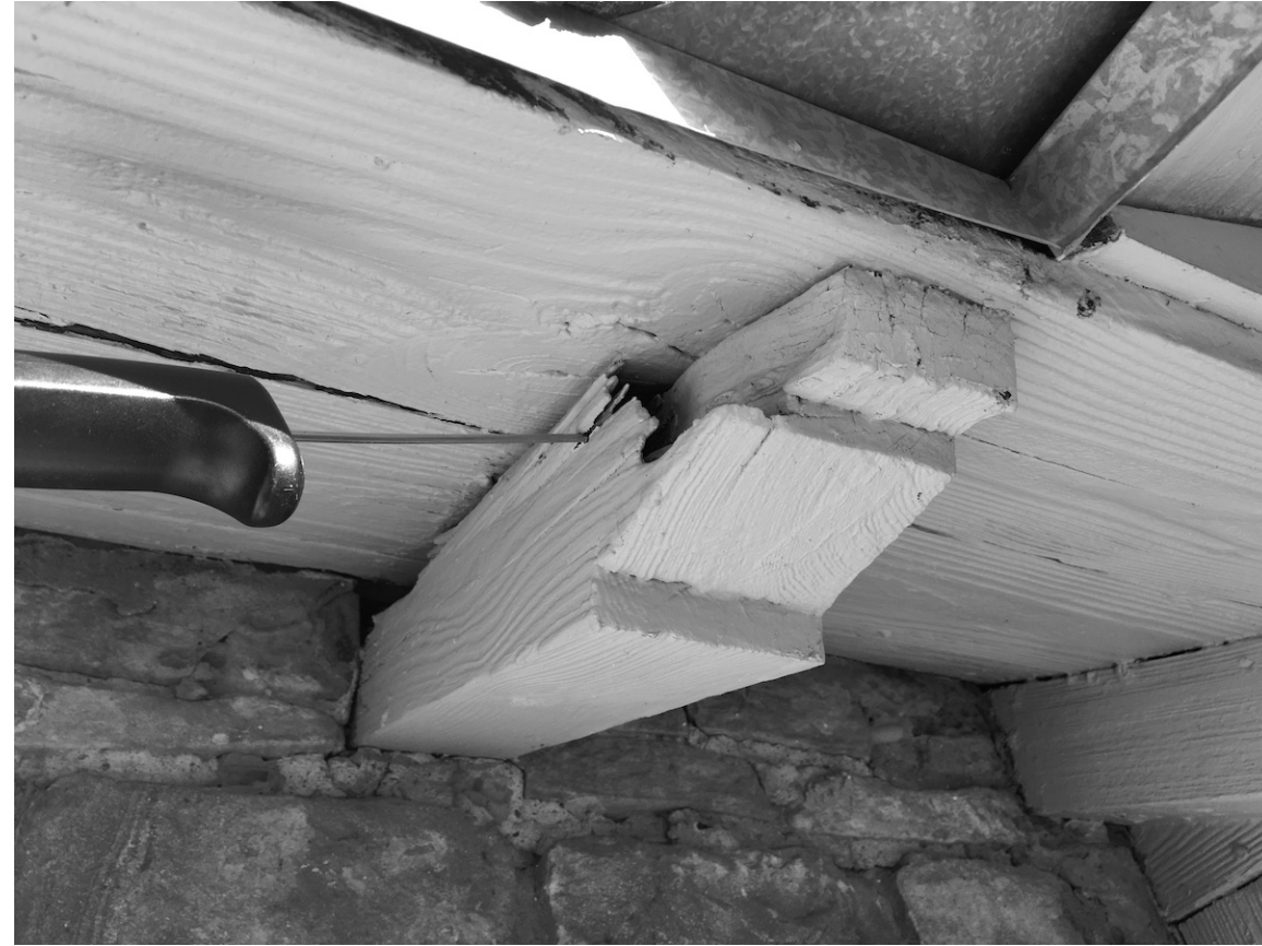
PHOTO 5 ROTTED RAFTER END
