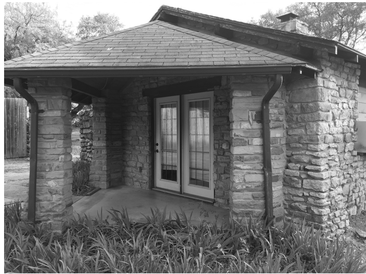
PHOTO 3 VIEW FROM NORTHWEST
