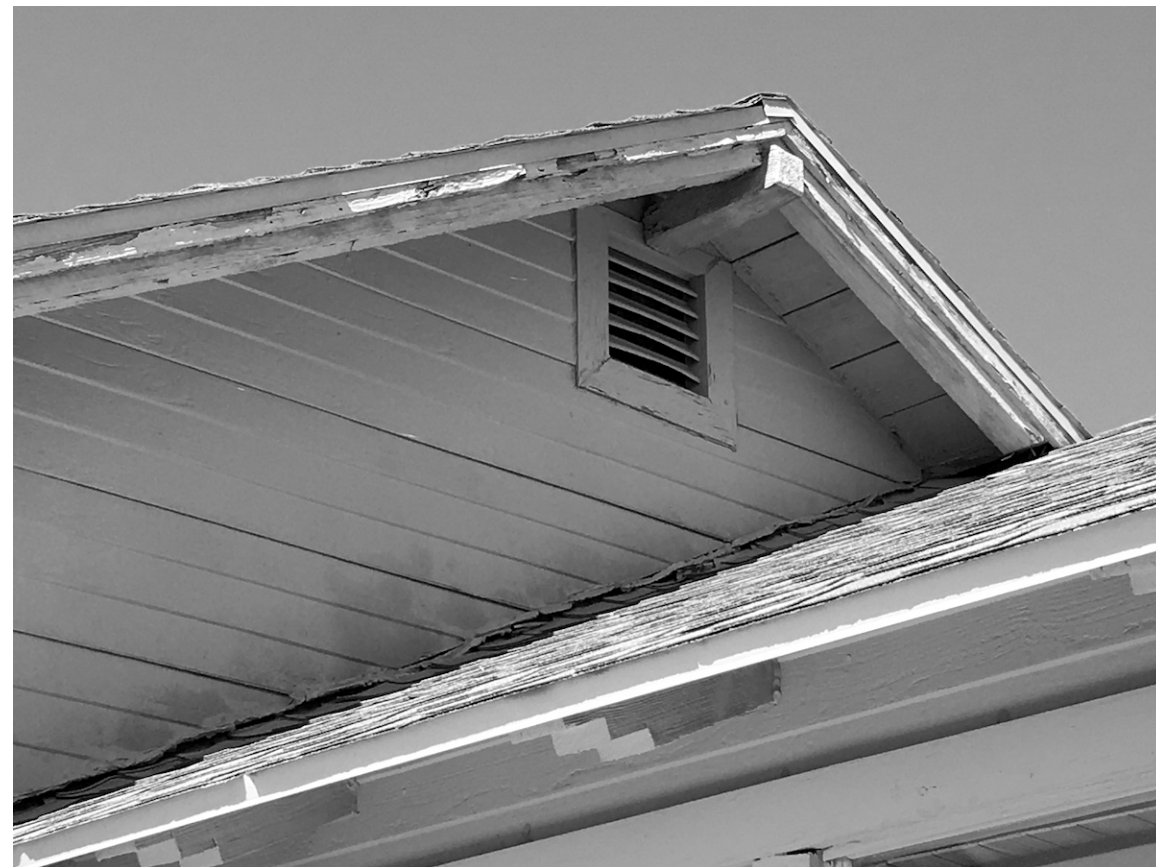
PHOTO 5 ROOF LOOKING NORTHWEST
