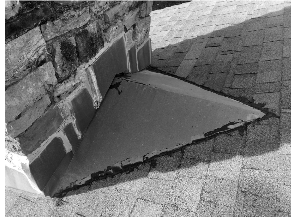
PHOTO 8 DETAIL AT CHIMNEY CRICKET
