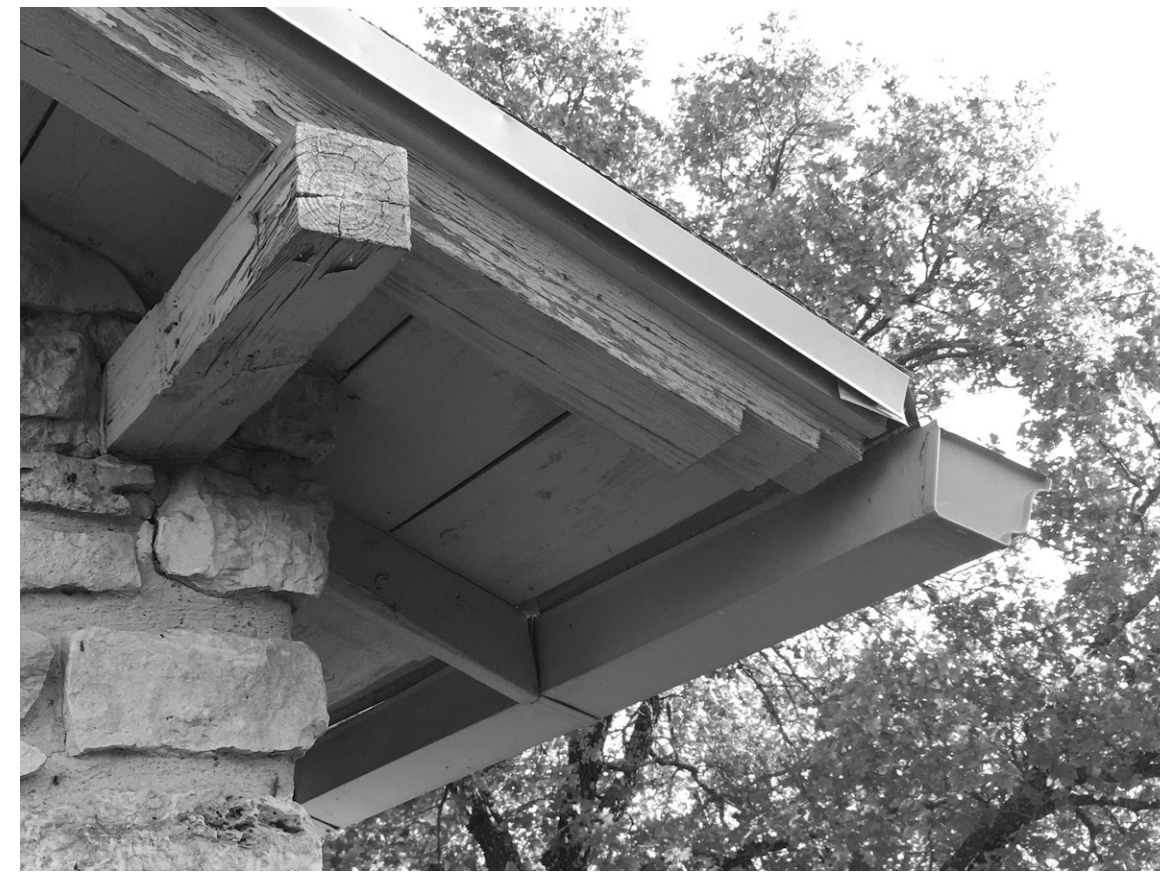
PHOTO 4 EAVE AND GUTTER AT SOUTHEAST
