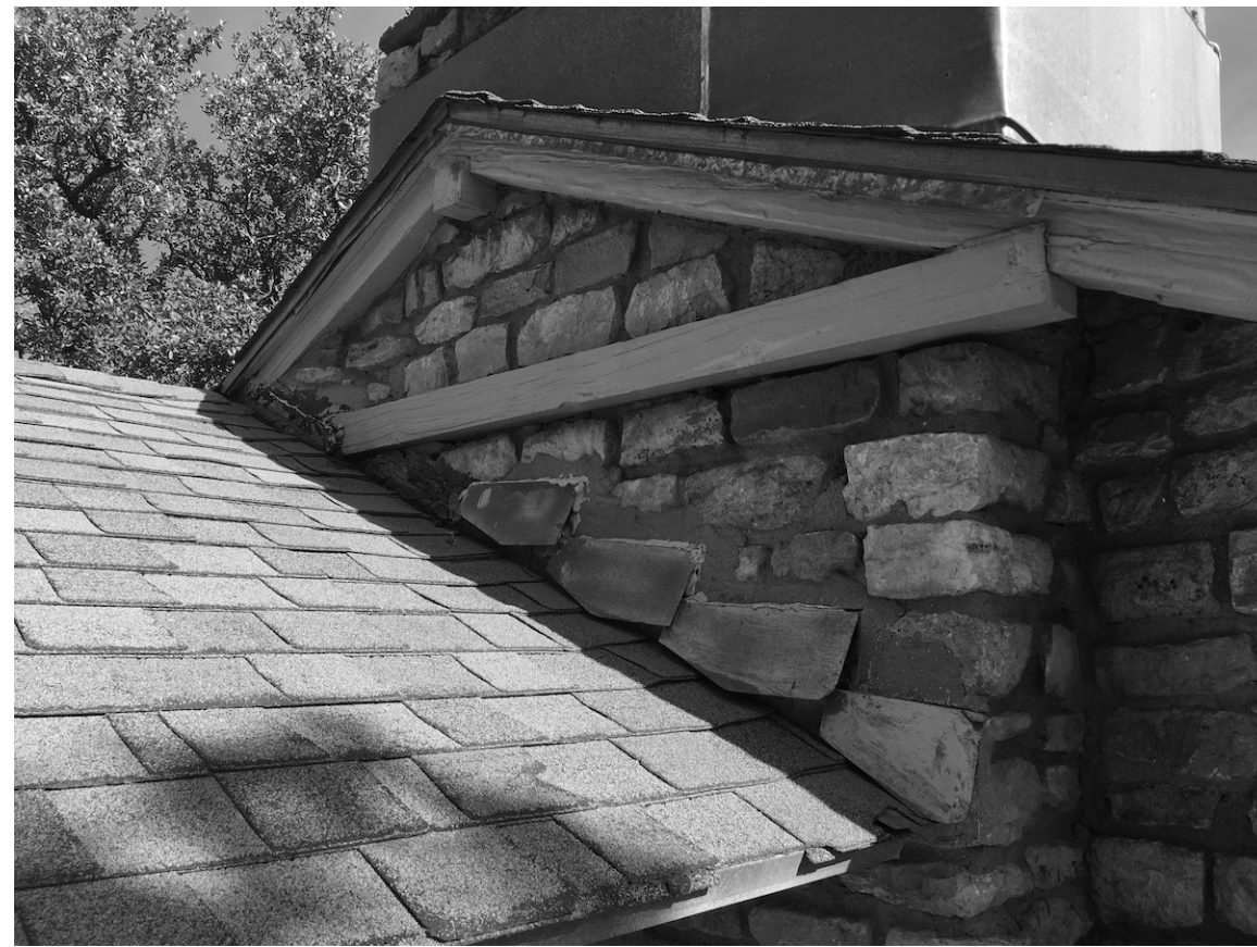
PHOTO 5 DETAIL AT WEST ELEVATION
