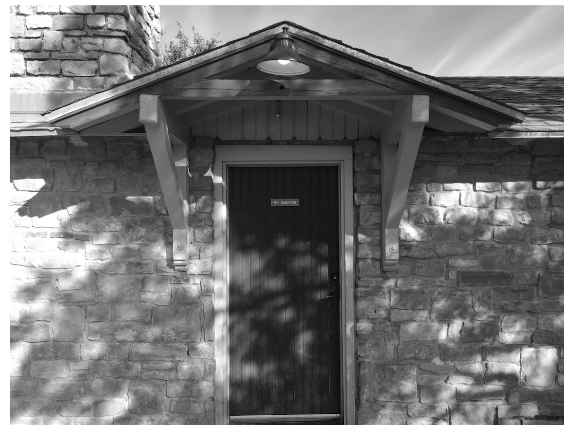
PHOTO 2 DETAIL OF ROOF OVER ENTRY
