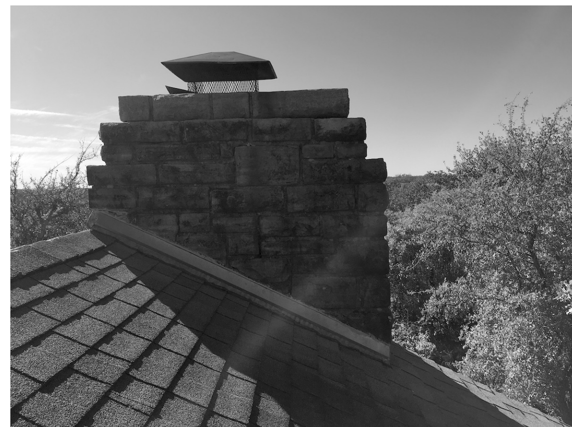
PHOTO 8 ROOF LOOKING WEST
