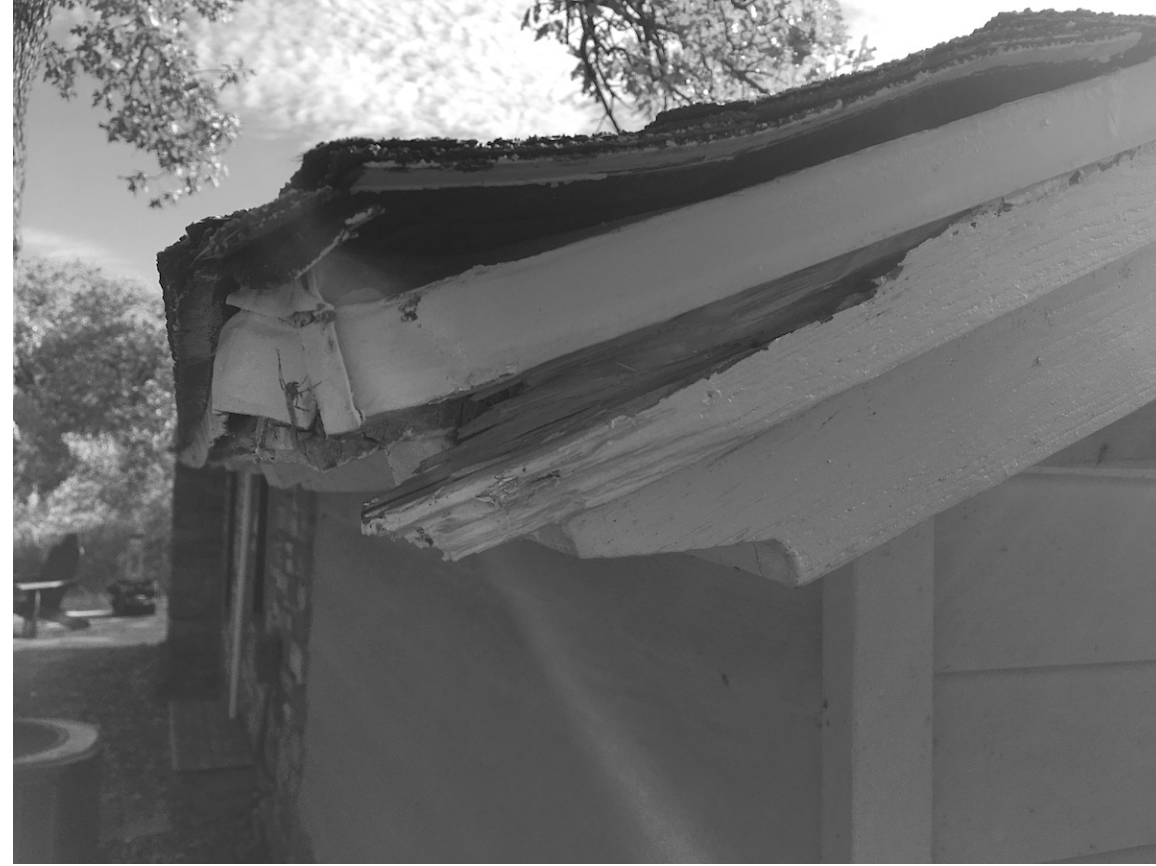
PHOTO 3 RAKE AT NORTHWEST CORNER
