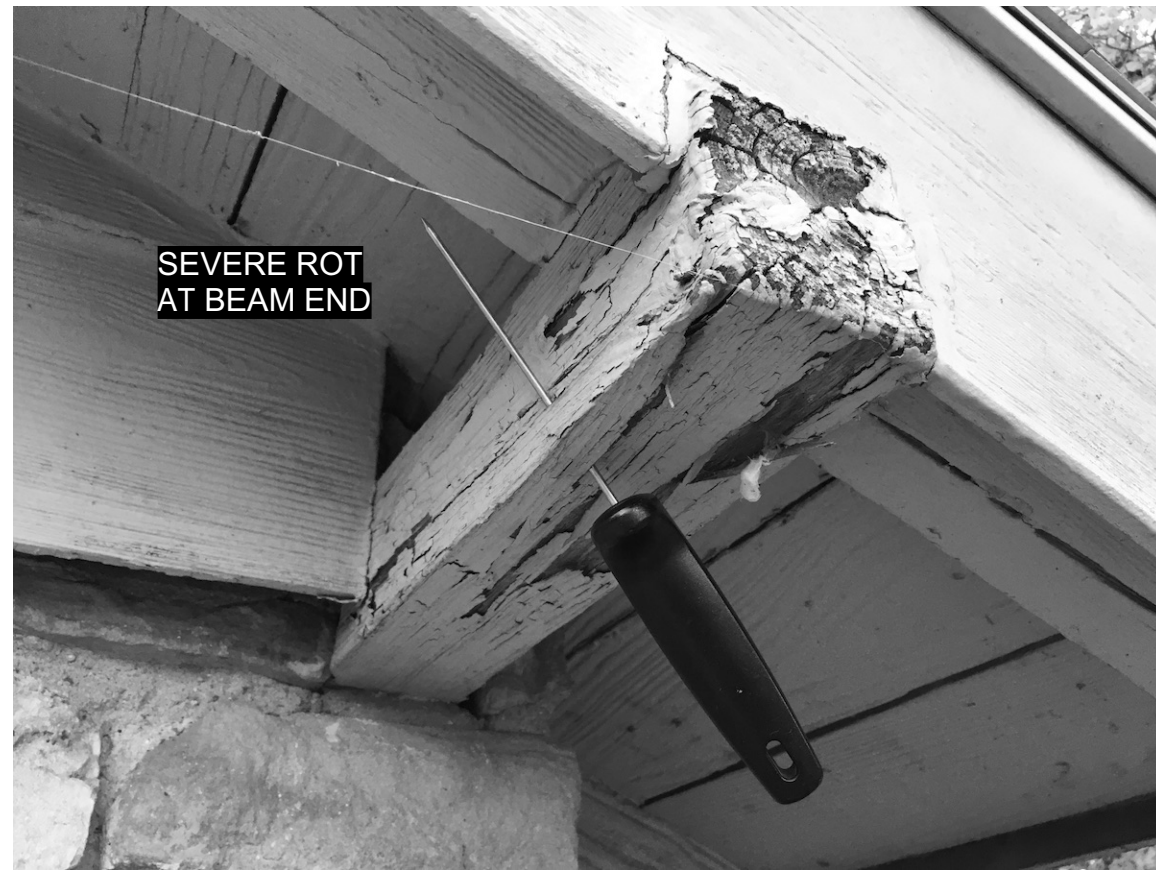
PHOTO 5 BEAM AT NORTHEAST CORNER
