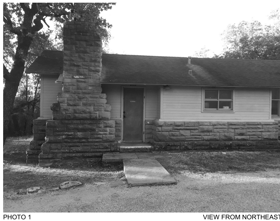
PHOTO 1 VIEW FROM NORTHEAST
