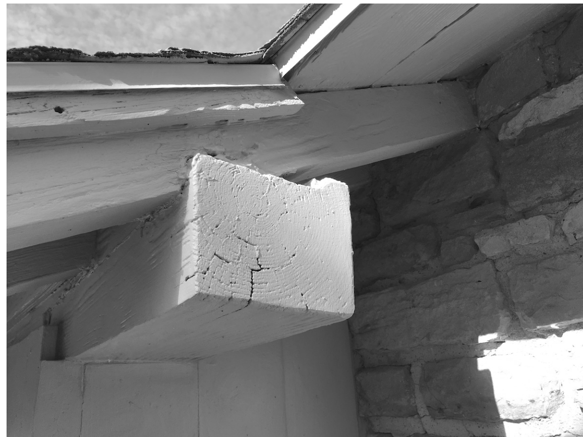
PHOTO 7 BEAM AT SOUTH WALL OFFSET
