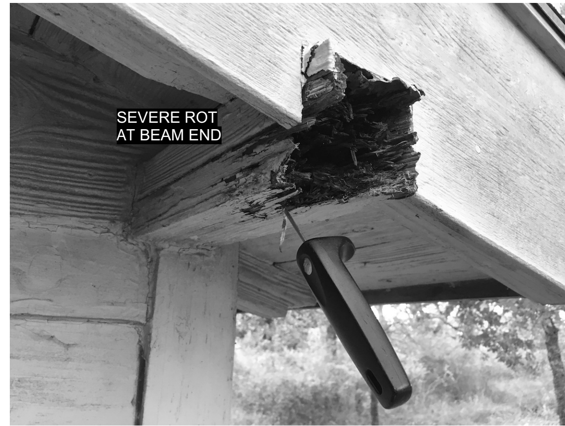
PHOTO 6 BEAM AT NORTH CORNER
