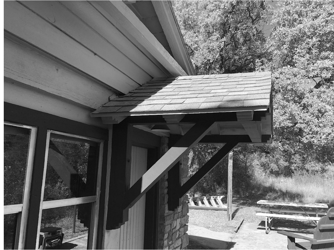
PHOTO 5 ROOF OVER ENTRY
