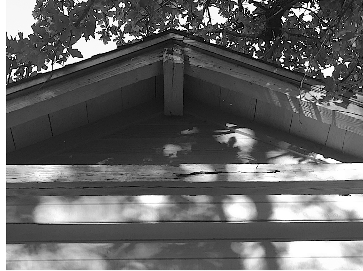
PHOTO 4 RAKE AT EAST ELEVATION
