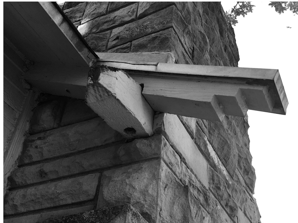
PHOTO 5 ROOF LOOKING SOUTHWEST
