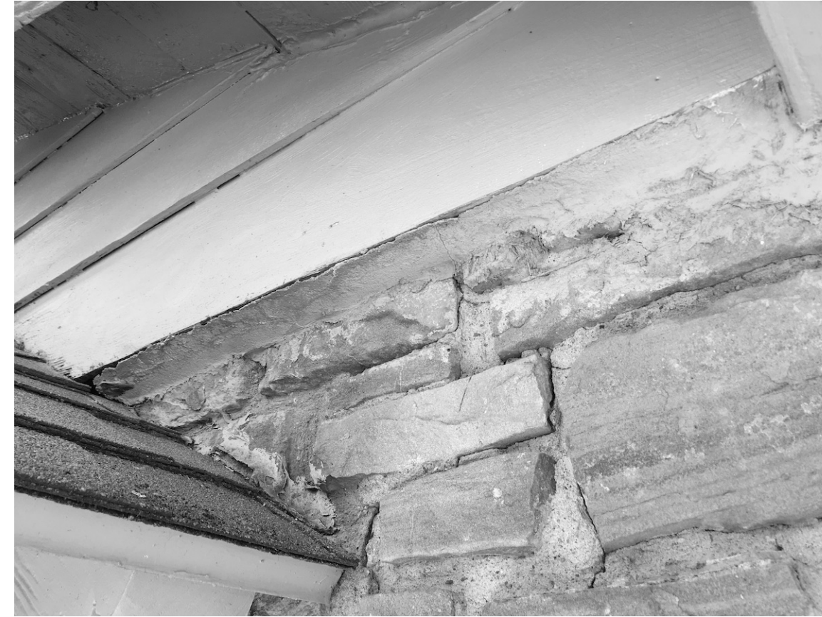
PHOTO 6 ROOF OVER ENTRY
