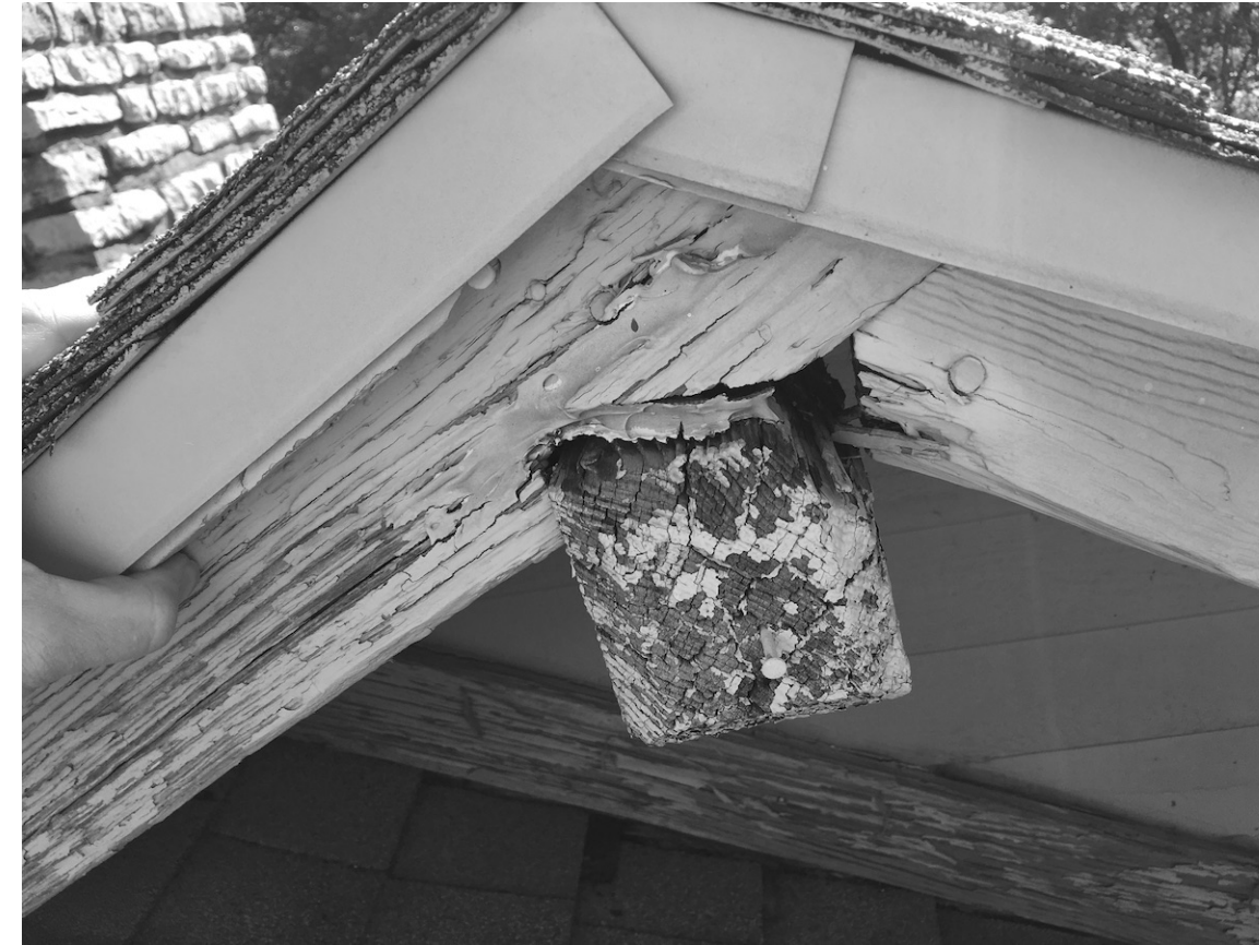
PHOTO 8 ROTTED WOOD AT WEST GABLE
