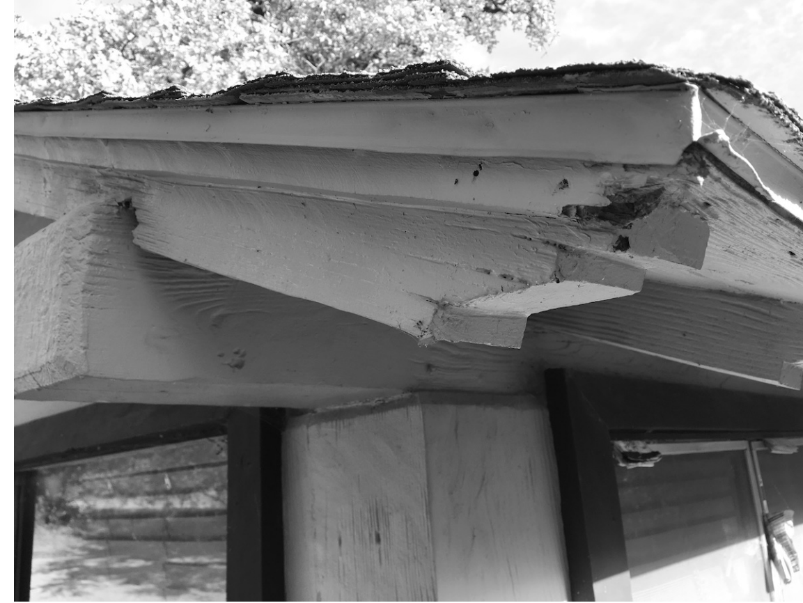
PHOTO 4 RAKE AT SOUTHWEST CORNER
