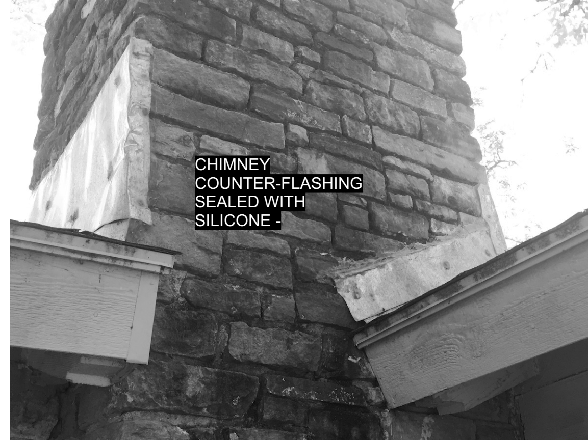
PHOTO 4 DETAIL AT CHIMNEY
