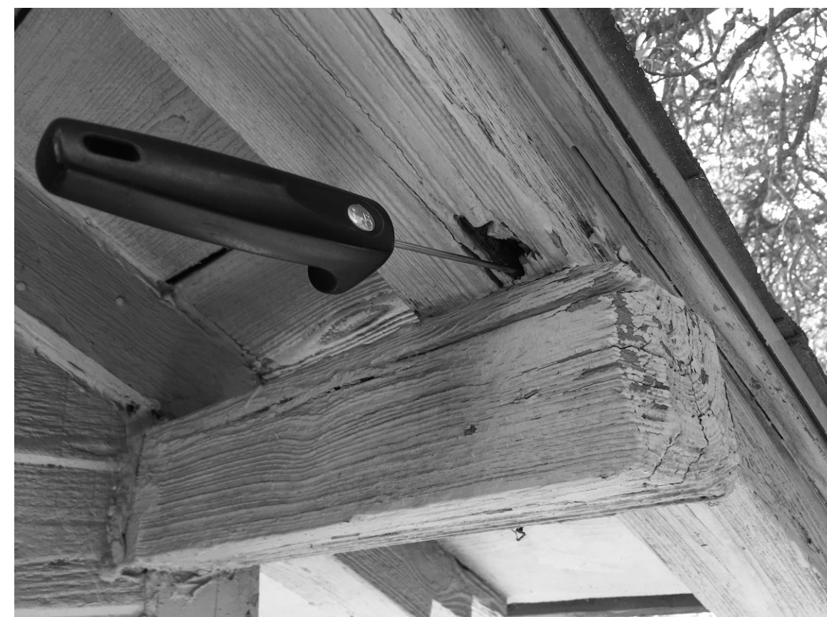
PHOTO 8 EAVE AT WEST ELEVATION
