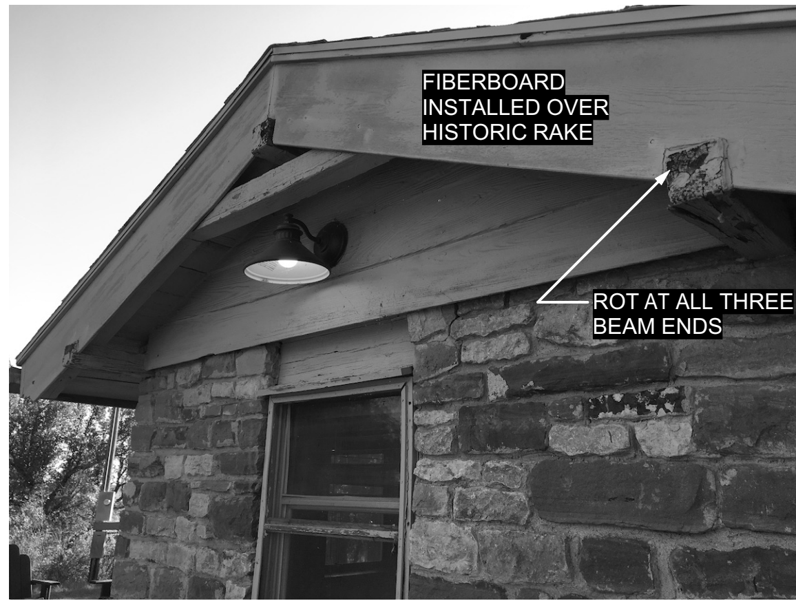
PHOTO 3 GABLE DETAIL AT EAST ELEVATION
