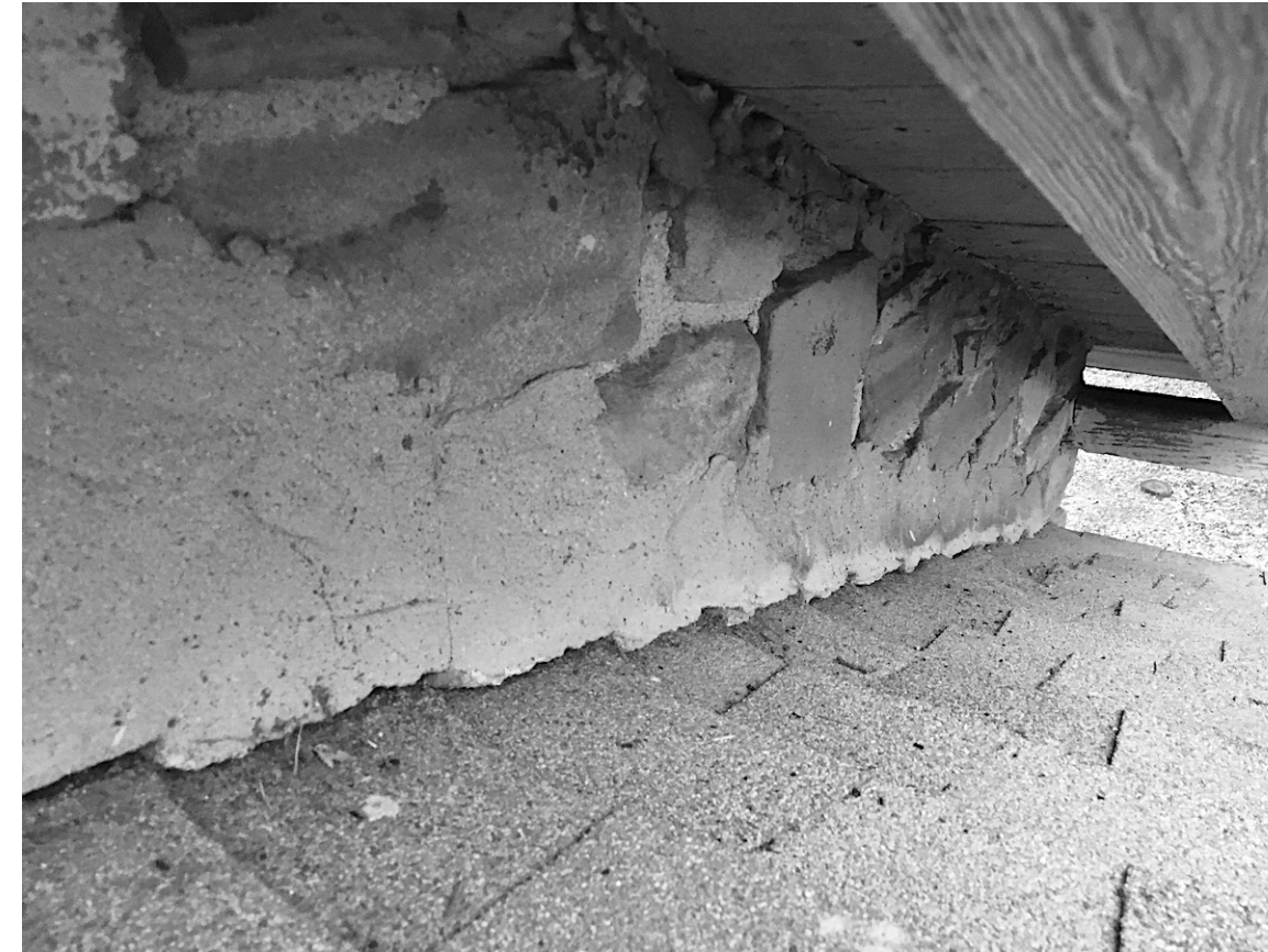
PHOTO 8 MORTARED FLASHING AT EAST LOWER ROOF
