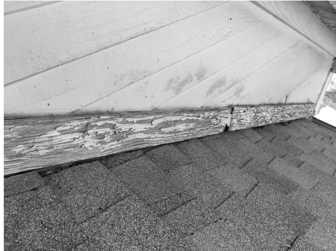
PHOTO 7 ROOF TERMINATION AT WEST GABLE
