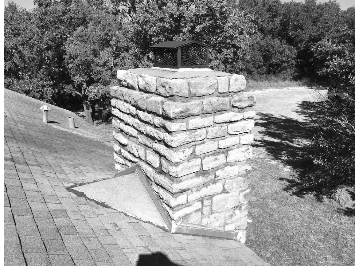
PHOTO 5 CHIMNEY AND CRICKET
