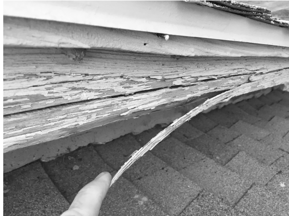
PHOTO 7 RAKE AT EAST GABLE
