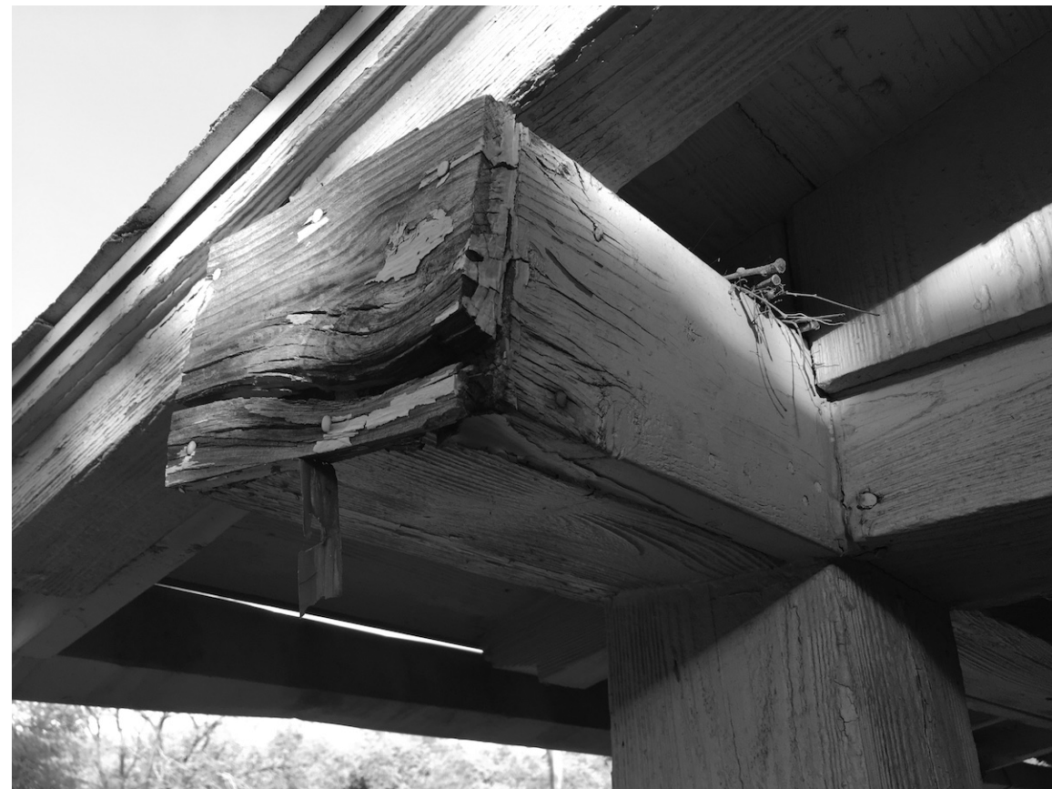
PHOTO 5 ROT AT BEAM NEAR ENTRANCE
