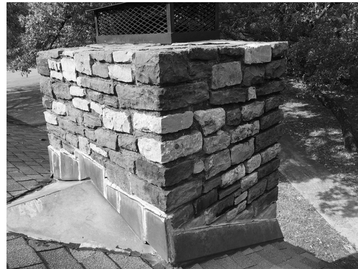
PHOTO 8 CHIMNEY AND CRICKET
