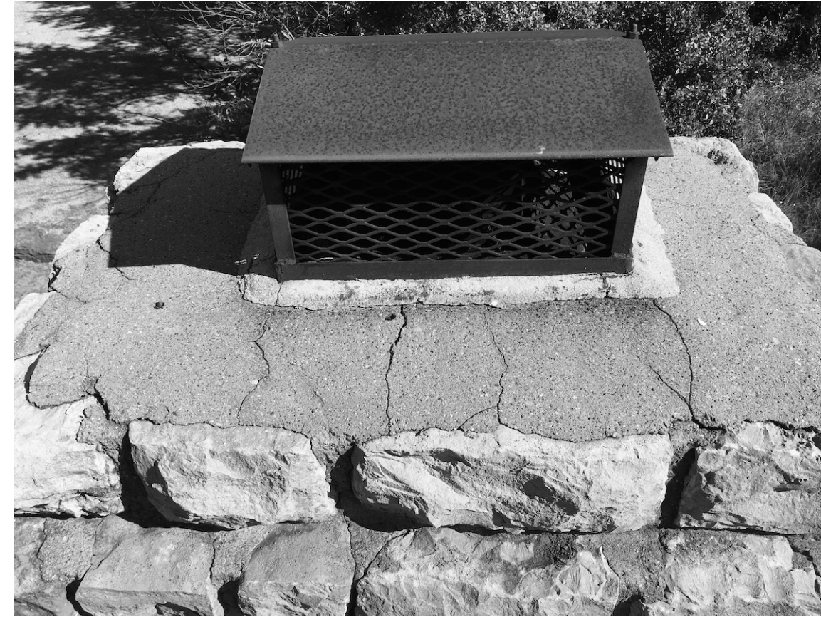
PHOTO 6 CRACKED MORTAR AT CHIMNEY
