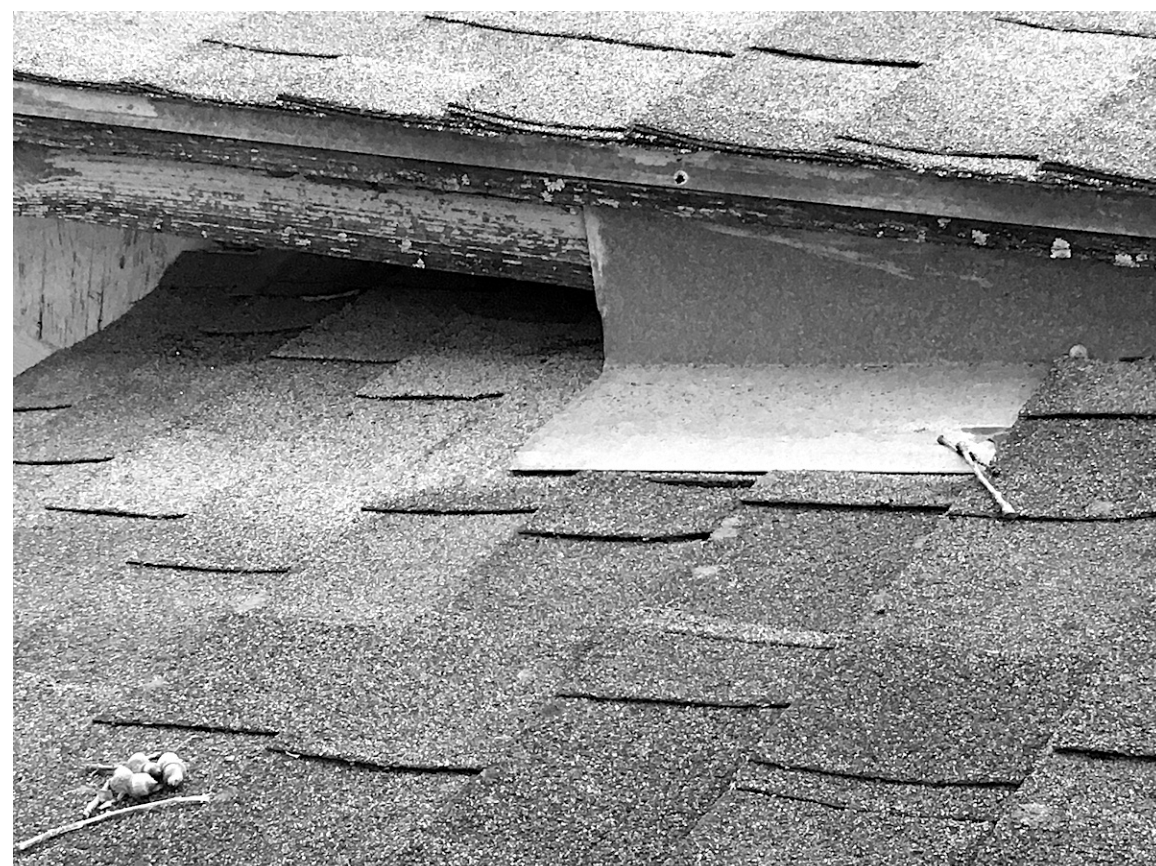
PHOTO 7 FLASHING AT ROOF OFFSET
