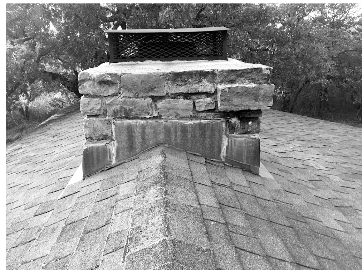
PHOTO 8 DETAIL OF CHIMNEY
