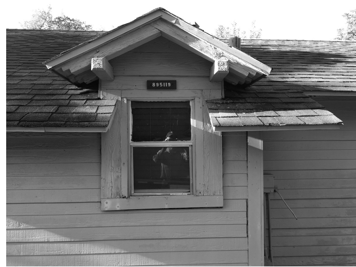
PHOTO 4 DETAIL AT NORTH ELEVATION WINDOW
