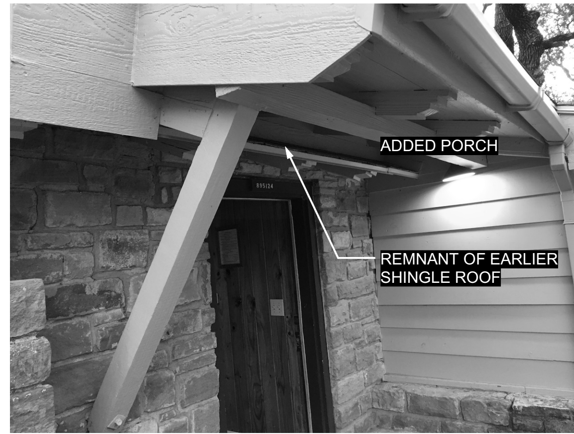
PHOTO 4 ADDED PORCH OVER ENTRANCE
