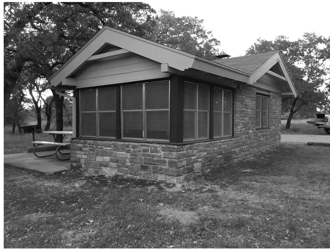
PHOTO 3 VIEW FROM SOUTHEAST
