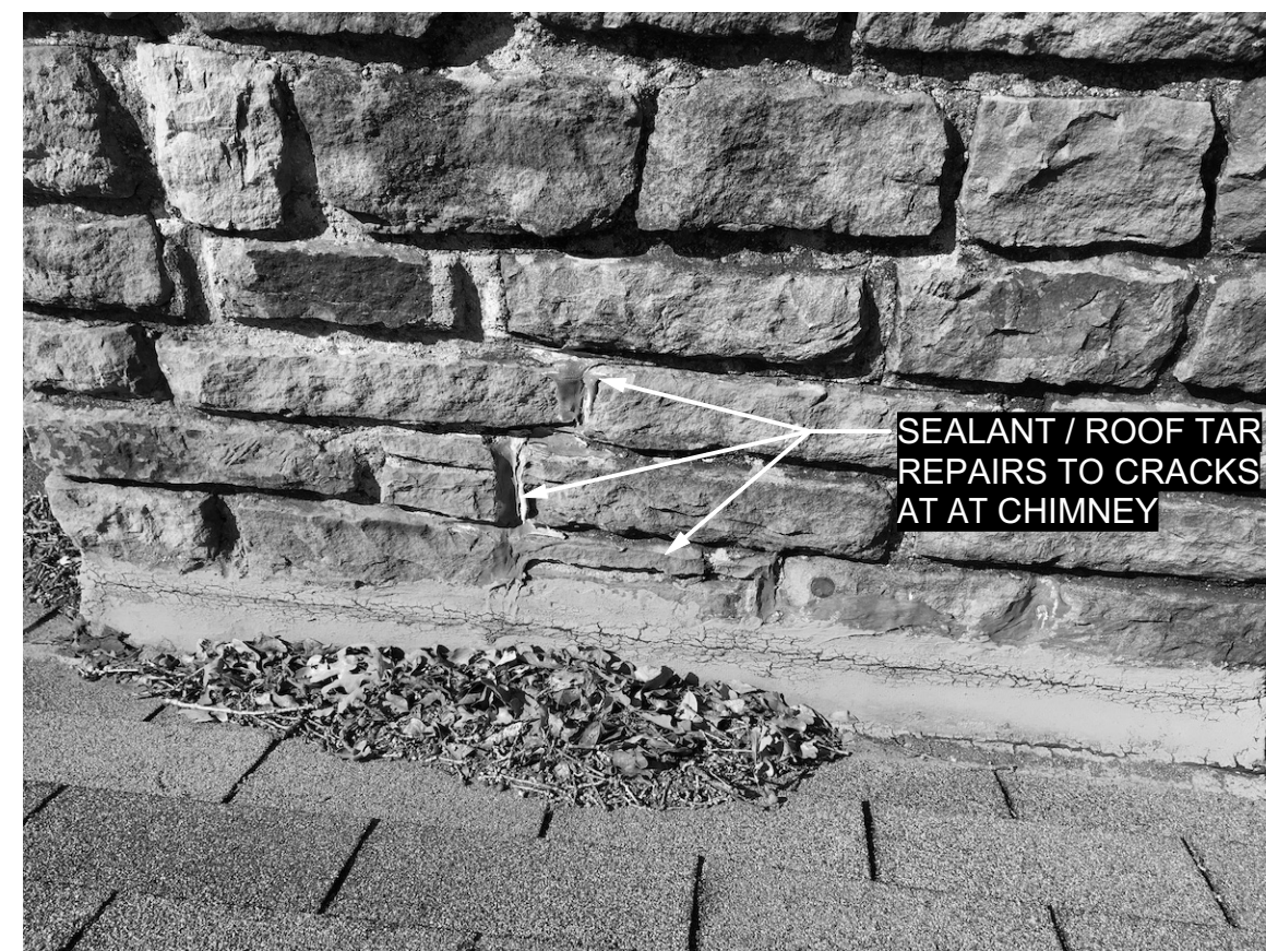
PHOTO 8 EAST SIDE OF CHIMNEY
