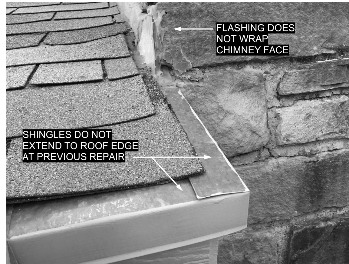
PHOTO 6 DETAIL AT CHIMNEY
