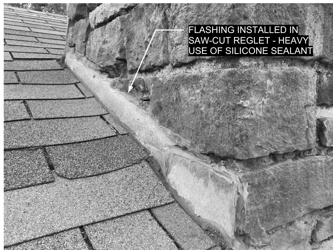
PHOTO 7 FLASHING AT CHIMNEY
