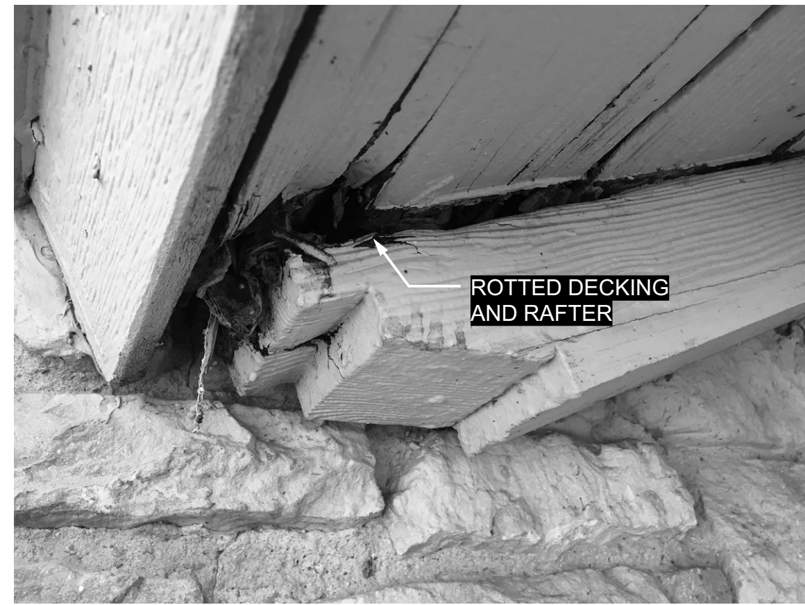
PHOTO 4 RAFTER TAIL AT CHIMNEY
