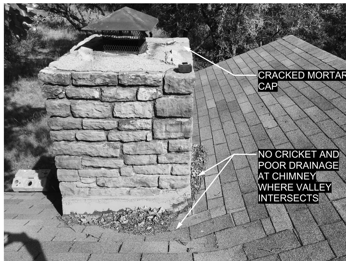
PHOTO 7 CHIMNEY LOOKING NORTH
