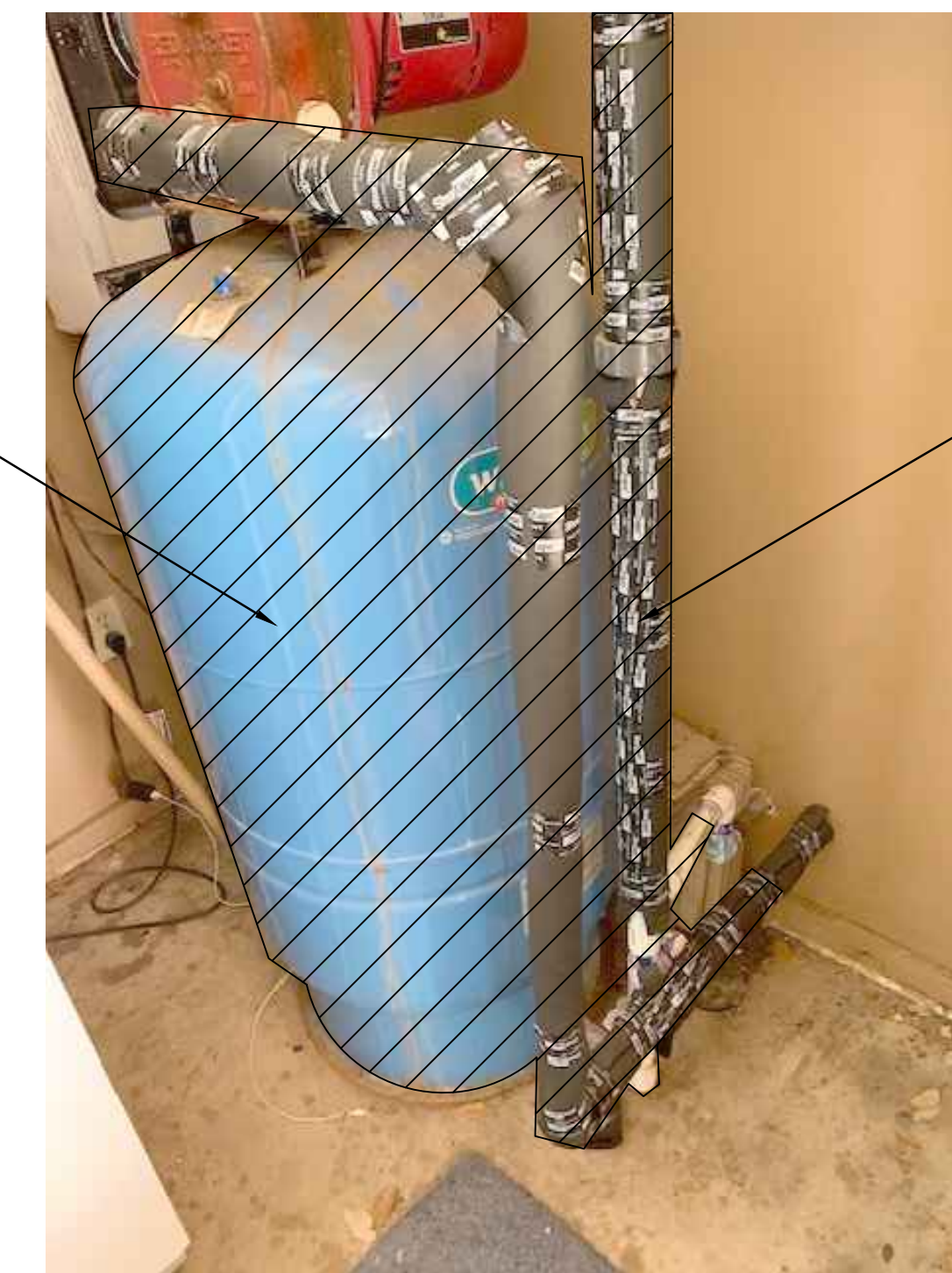
3 99-C503 99-C503 SCALE: NONE EXISTING RESIDENCE BOOSTER PUMP DETAIL
