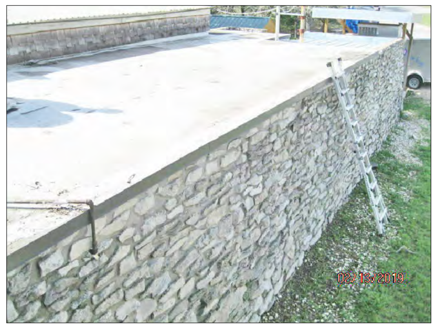
B ROOF VIEW
