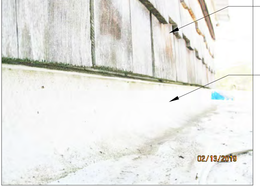
F VIEW OF SIDEWALL BASE
