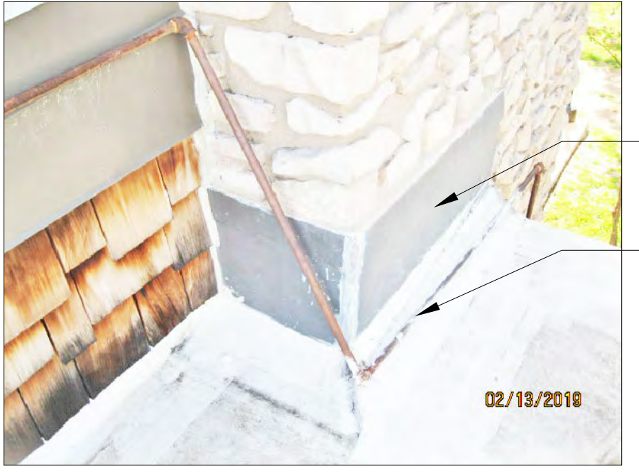
J VIEW AT EXISTING CHIMNEY FLASHING
