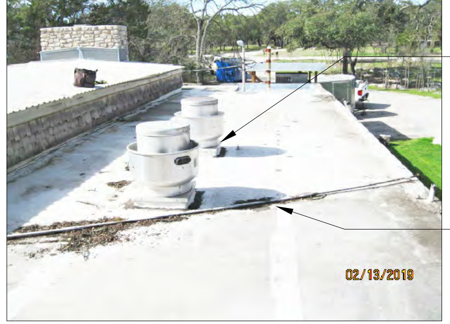
G ROOF VIEW AT EXHAUST FANS
