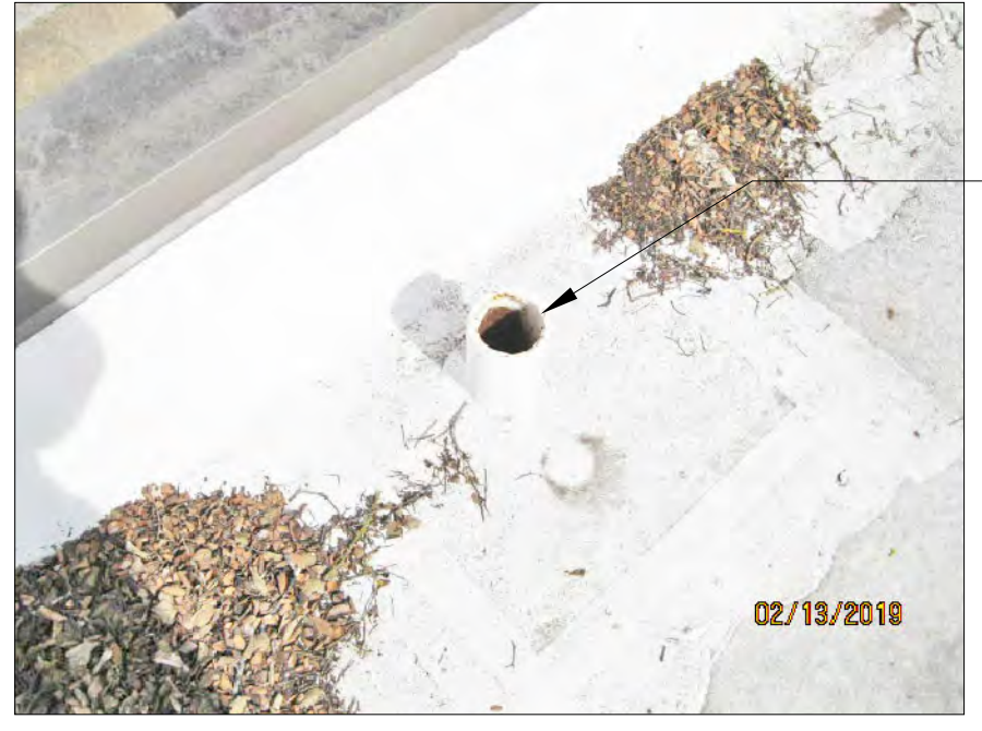
K VIEW AT ROOF PENETRATION
