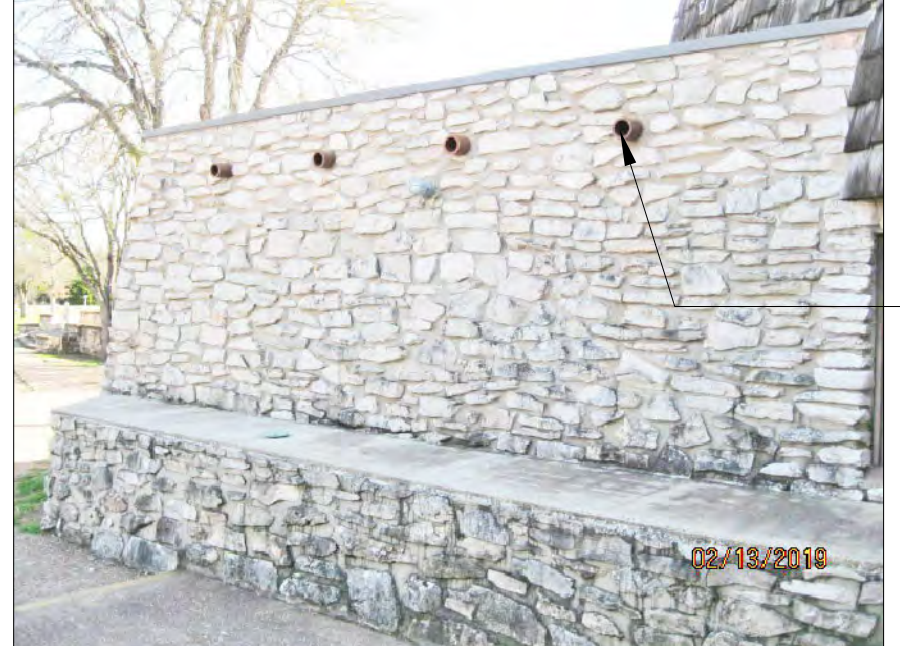
C VIEW AT EXISTING SCUPPER DRAINAGE PIPES
