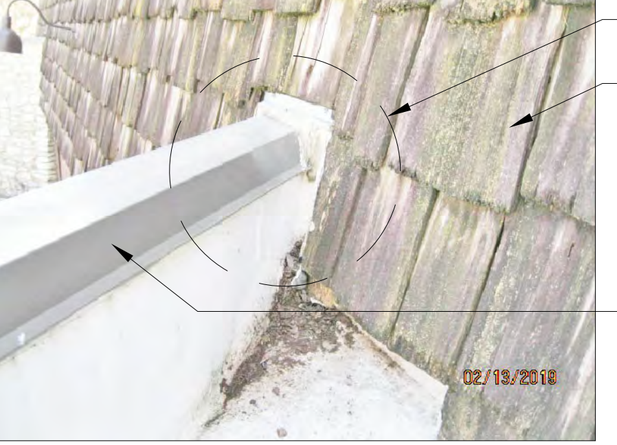
E VIEW AT PARAPET WALL END
