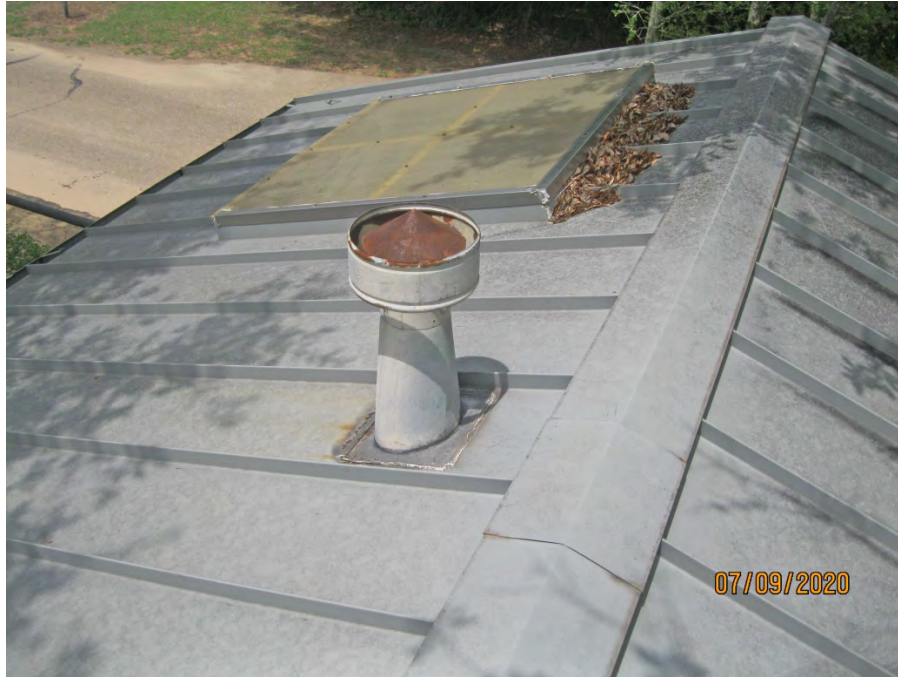
E. Detail View at Existing Roof Penetration
