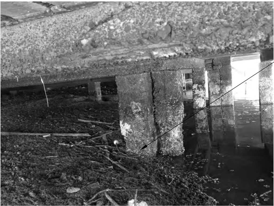
06 DETERIORATED CONCRETE COLUMNS NO SCALE
