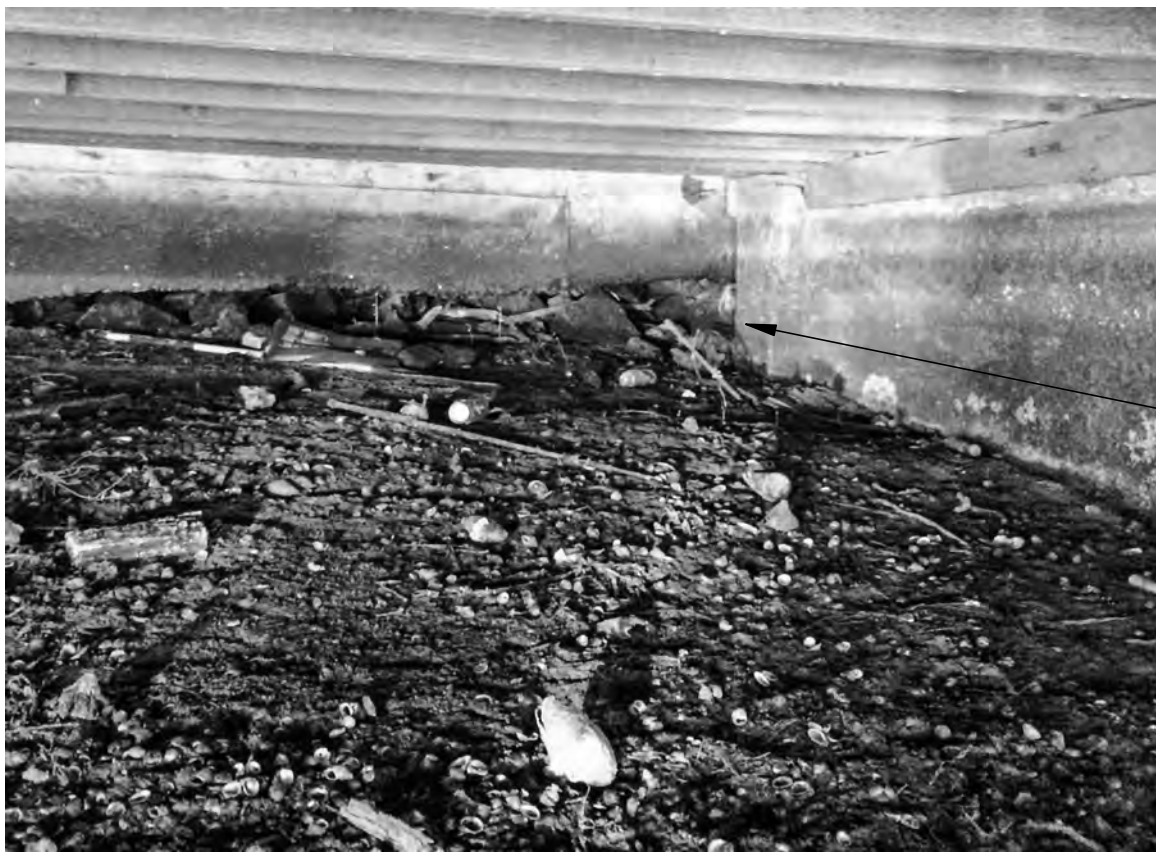
02 EROSION AT CONCRETE WALL NO SCALE
