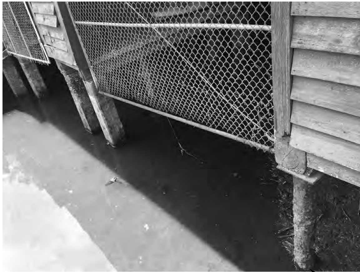
05 CORRODED STEEL PIPE COLUMN NO SCALE
