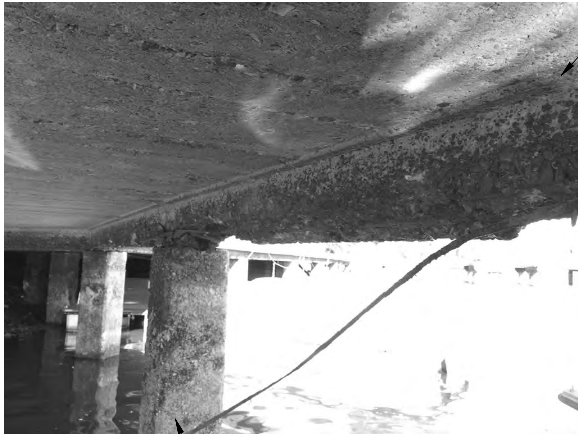
01 DETERIORATED CONCRETE BEAM NO SCALE
