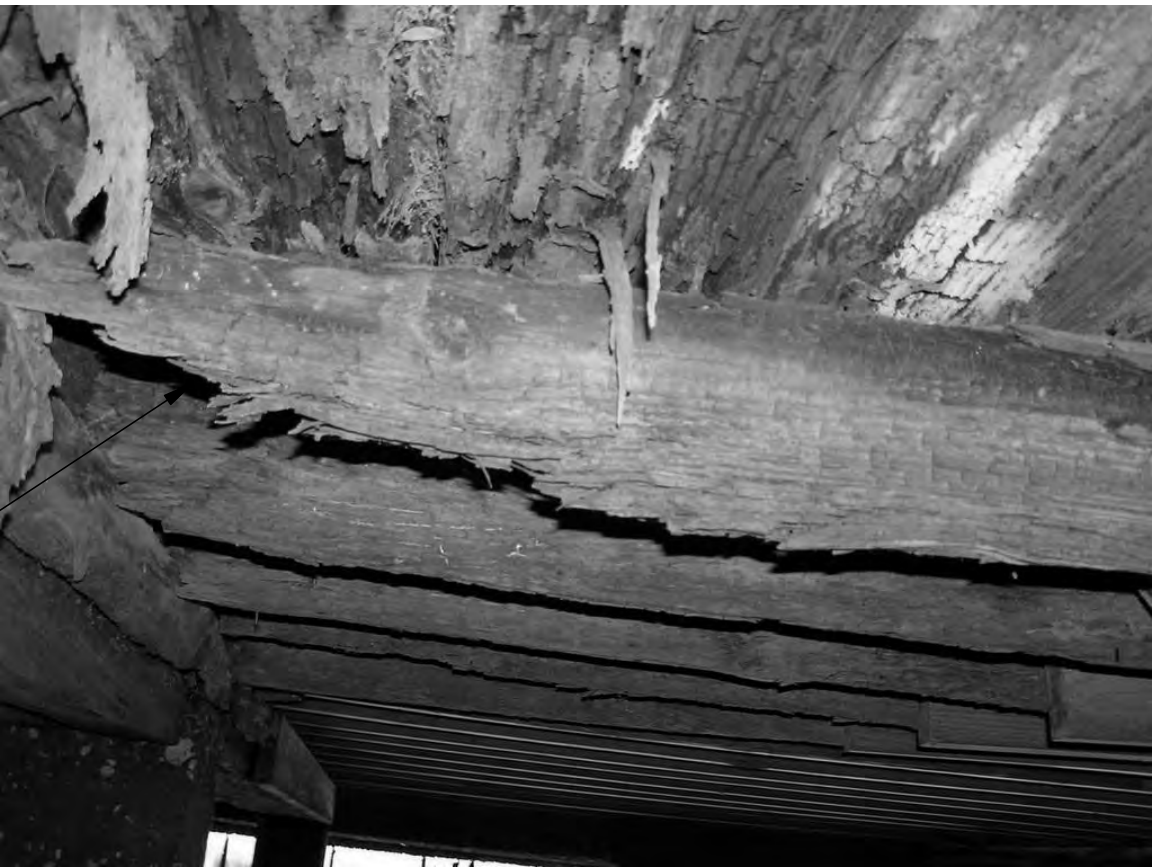
04 DETERIORATED WOOD JOISTS & DECK NO SCALE
