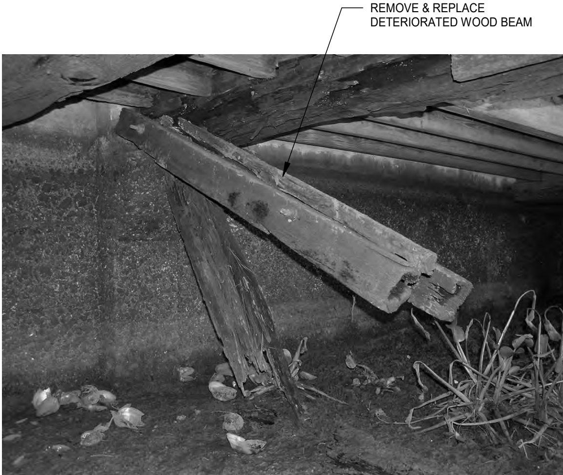
03 DETERIORATED WOOD BEAM NO SCALE
