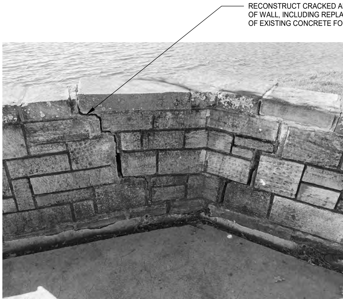
09 CRACKED & SHIFTED RETAINING WALL NO SCALE
