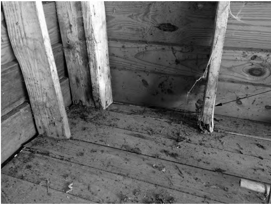
07 DETERIORATED WOOD WALL STUDS NO SCALE
