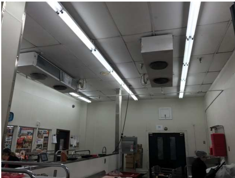
PHOTO 8 - 2' X 4' SHEETROCK CEILING TILE
