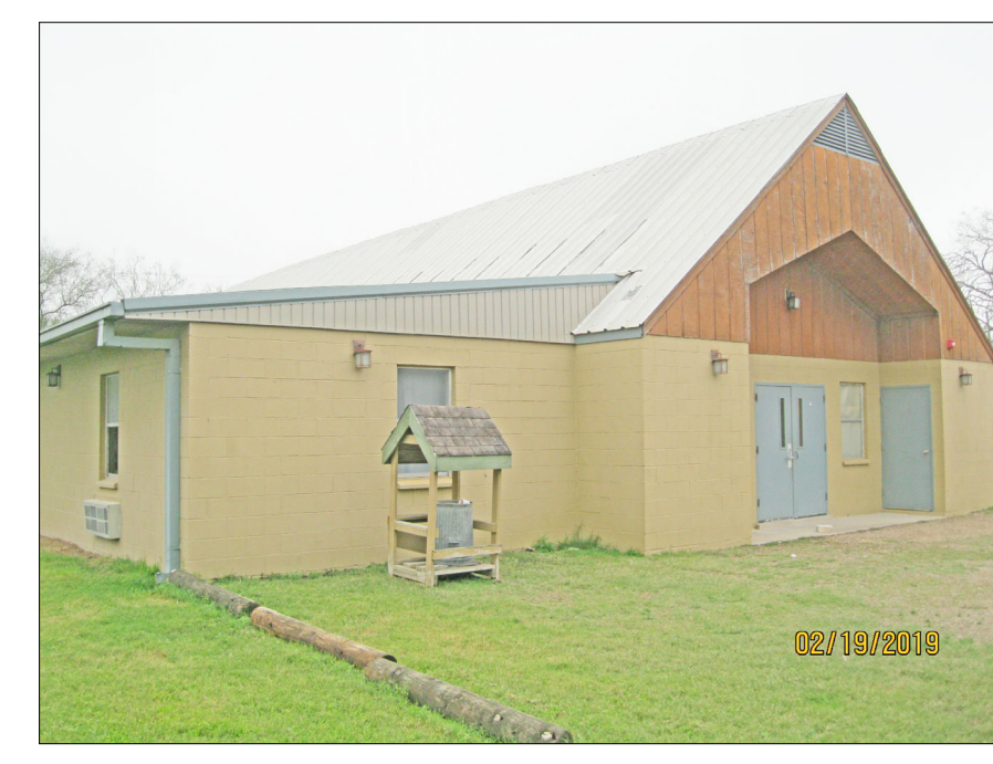
B EAST VIEW OF BUNKHOUSE
