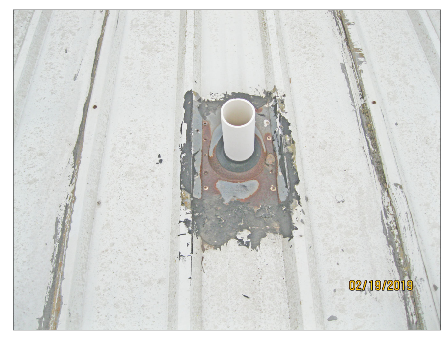
E ROOF VIEW AT EXISTING VENT THROUGH ROOF
