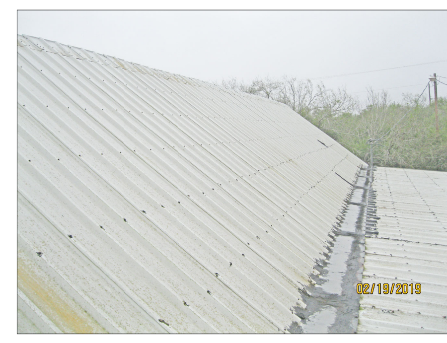
D ROOF VIEW AT SLOPE TRANSITION FLASHING
